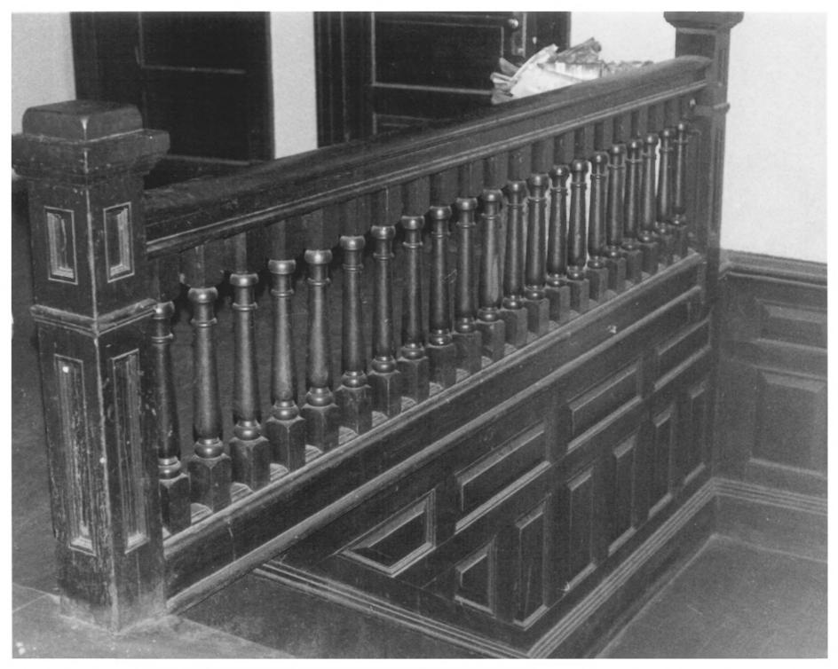
11 of 14 Detail of stairway paneling and railing.
