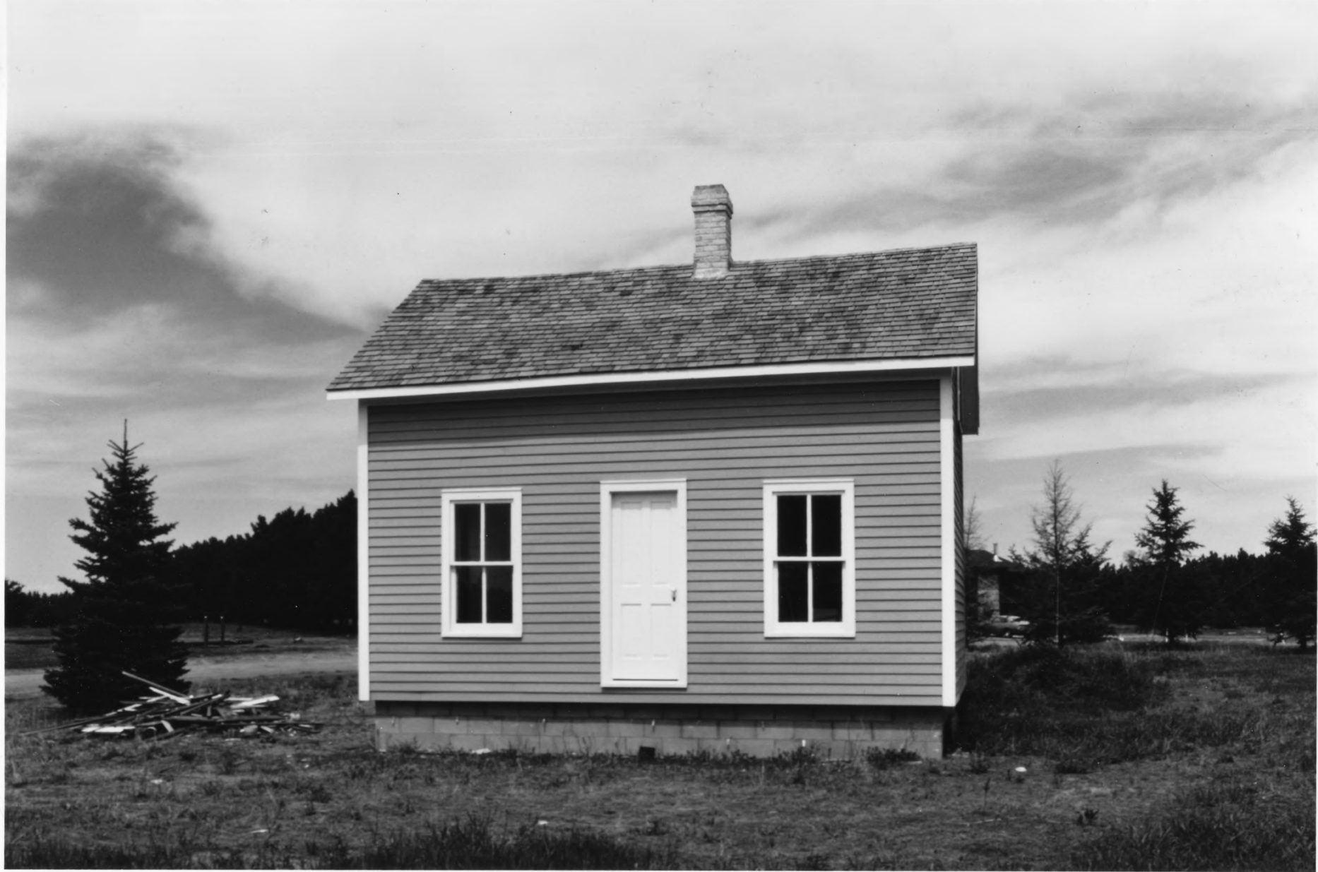
FOX, HERBERT M., HOUSE VICINITY OF BECKER, BECKER TWP., SHERBURNE CO., MINNESOTA #49004
