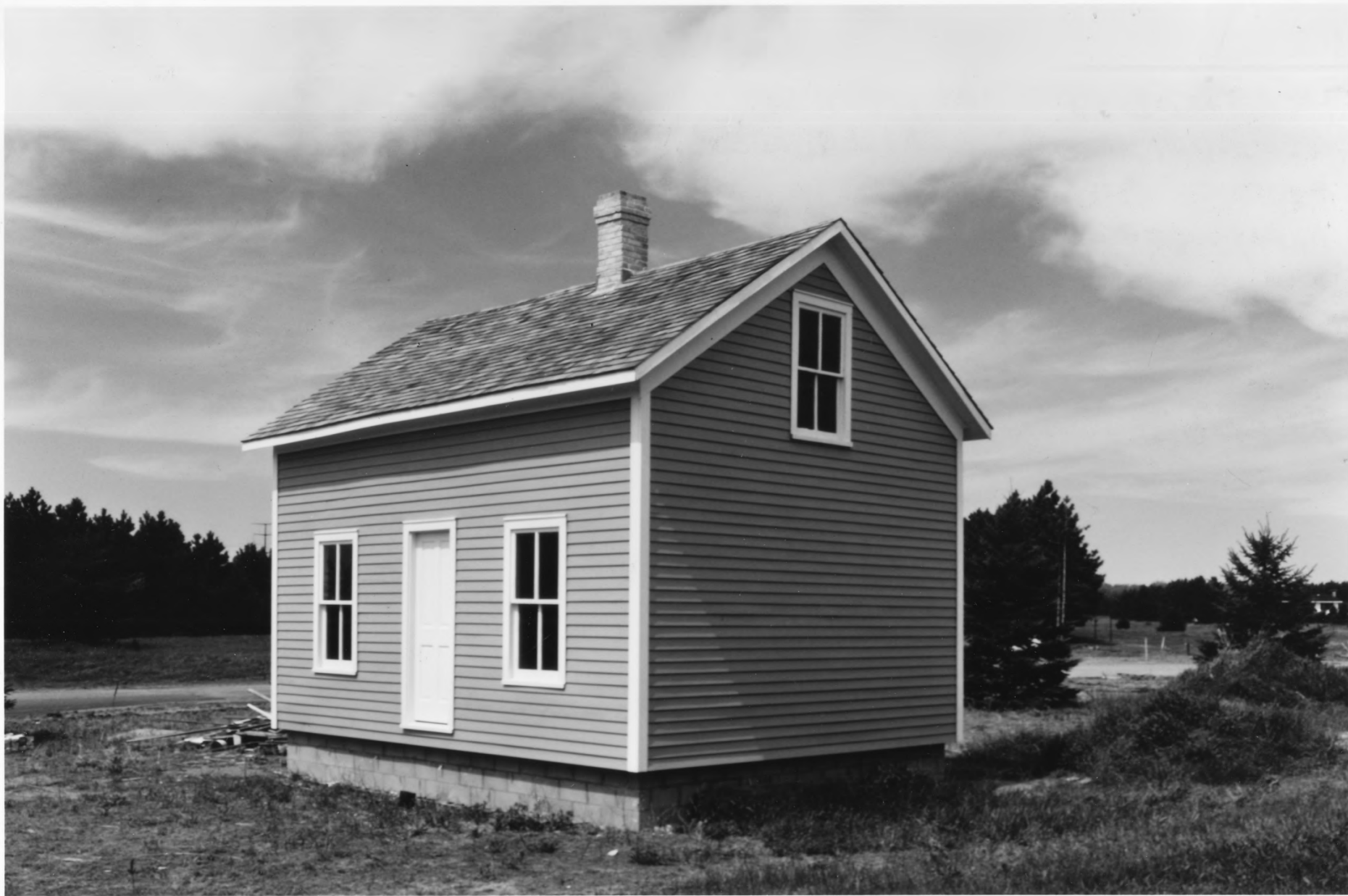
FOX, HERBERT M., HOUSE VICINITY OF BECKER, BECKER TWP., SHERBURNE CO., MINNESOTA #49005
