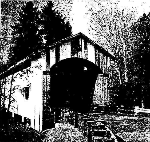
Lane County repaired the damaged needle beam at the Wendling Bridge (37-20-36). The old structure was enforced by a 4x6 crutch when the 1990 safari visited.
