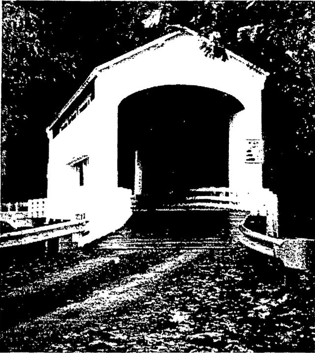
Once again, traffic flows through the Wildcat (37-20-04) covered bridge, just off Highway 126 west of Eugene in Lane County. Crews worked during the summer to complete the rehabilitation which included a major overhaul of the structure. The roof, decking, bracing and other repairs makes the span look new again. A number of members reported that the bridge was reopened, and a trip to the bridge proved them right. The Wildcat span glows from the new wood and fresh paint.
