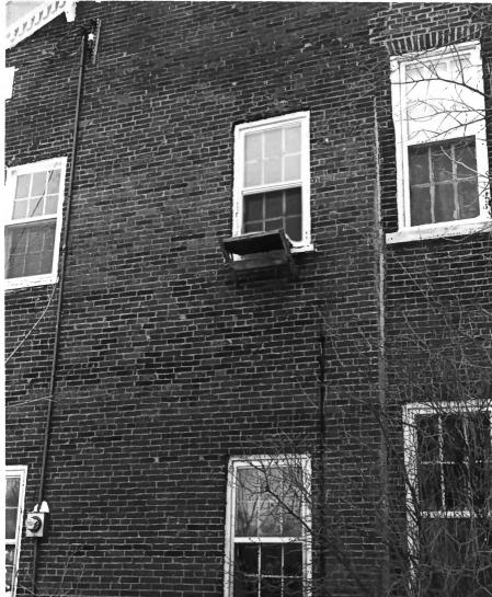
Charles Berryhill House MAY 3 | 1979 # 30K Iowa City, Johnson Co., Iowa Credit: M.H. Bowers Date: January 1979 APR 2 5 1979 Neg. at: SHPO, Iowa City IA View: closeup west elevation, showing original windows (L) and windows added during enlargement /
