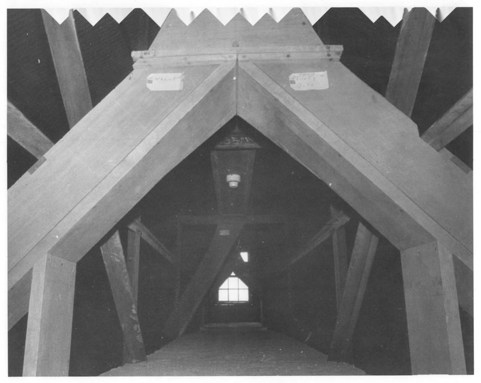
View looking west down catwalk over silos. Note chutes which took grain from overhead screw conveyor to silos below.
