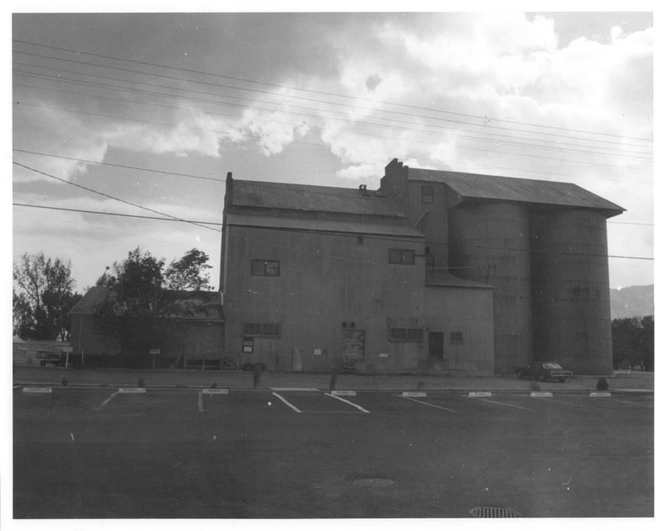
North-side view of mill showing corrugated sheet metal sheds attached to the main brick structure, and the four 45'high by 23'diameter steel grain-storage silos. The V&T Railroad served the mill from this side.
