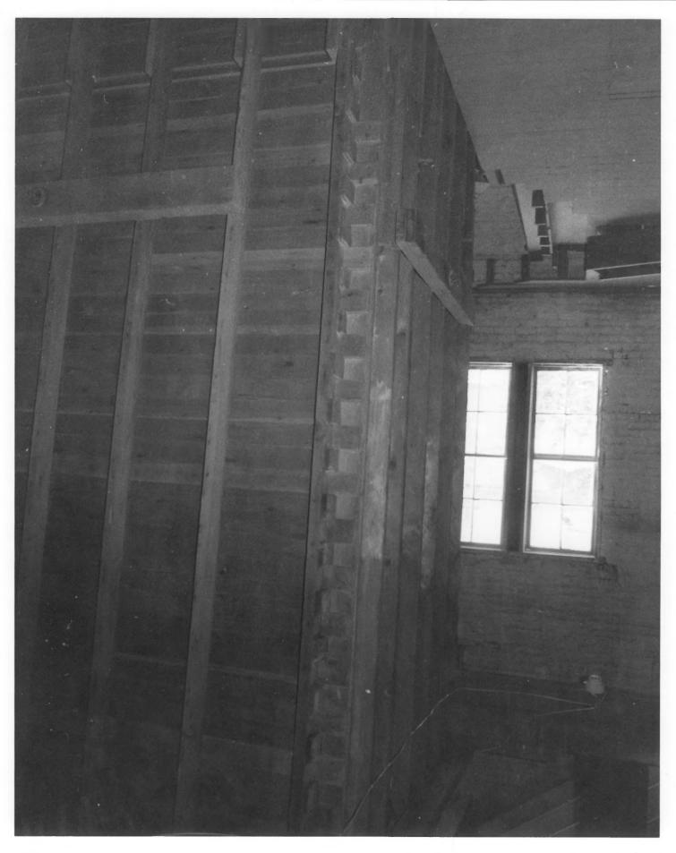
Third-floor pine bin in middle of floor with intricate carpentry. Floor in background partially removed in 1942 to accomodate metal molasses tanks installed on second floor. Windows facing east.
