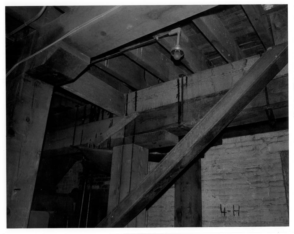
View toward ceiling of first floor showing extra support posts and beams installed to support molasses tanks on second floor when mill was converted to a feed mill in 1942. Shown is east brick wall of main structure and one of many pine grain chutes (running diagonally top right to bottom middle).
