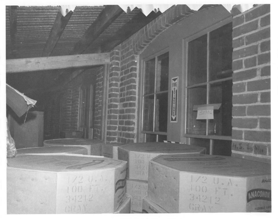
South-side (U.S.Hwy 395) one-story dock area (now enclosed) with corrugated sheet metal roof. South-side brick wall contains large windows looking into first-floor main room of brick structure. (Boxes are temporarily stored for Bently Nevada Corp).
