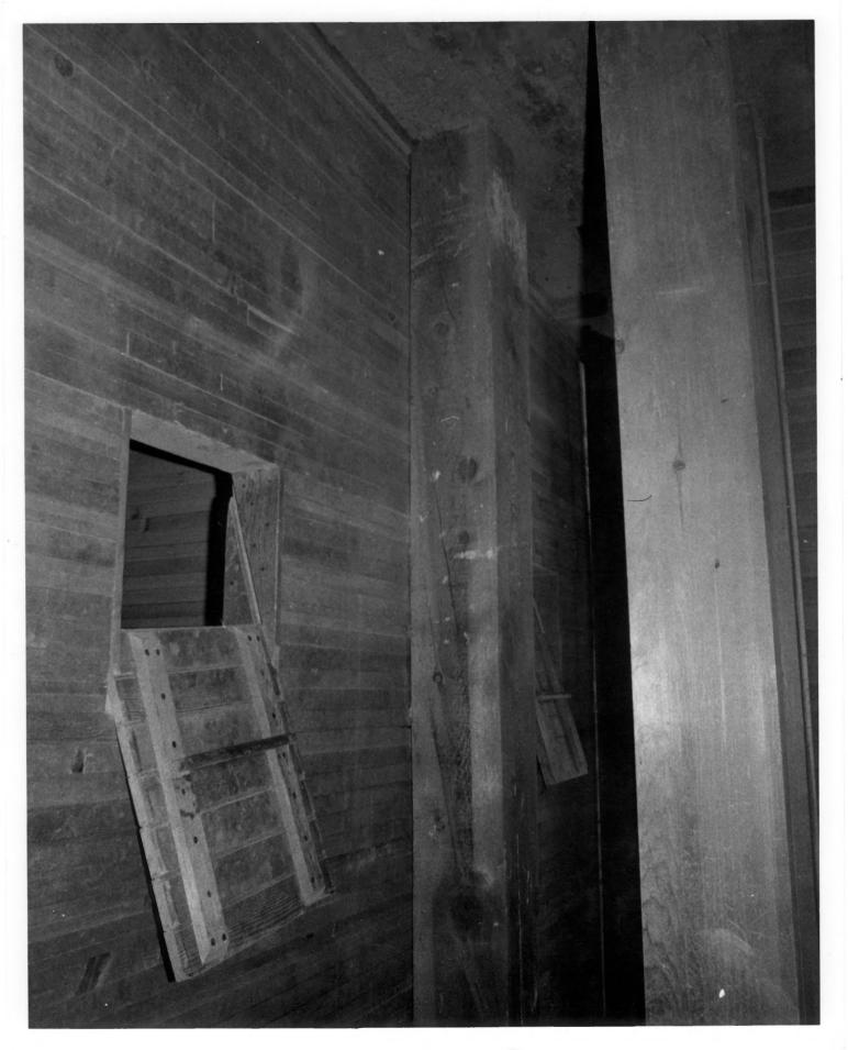
Second-floor view of pine grain bin (one of four against west brick wall) which extends up through third floor. Note use of fullmeasure 2" by 6" pine stacked flat to form bin walls and the smooth wood surface inside the bin created by constant flow of grain.
