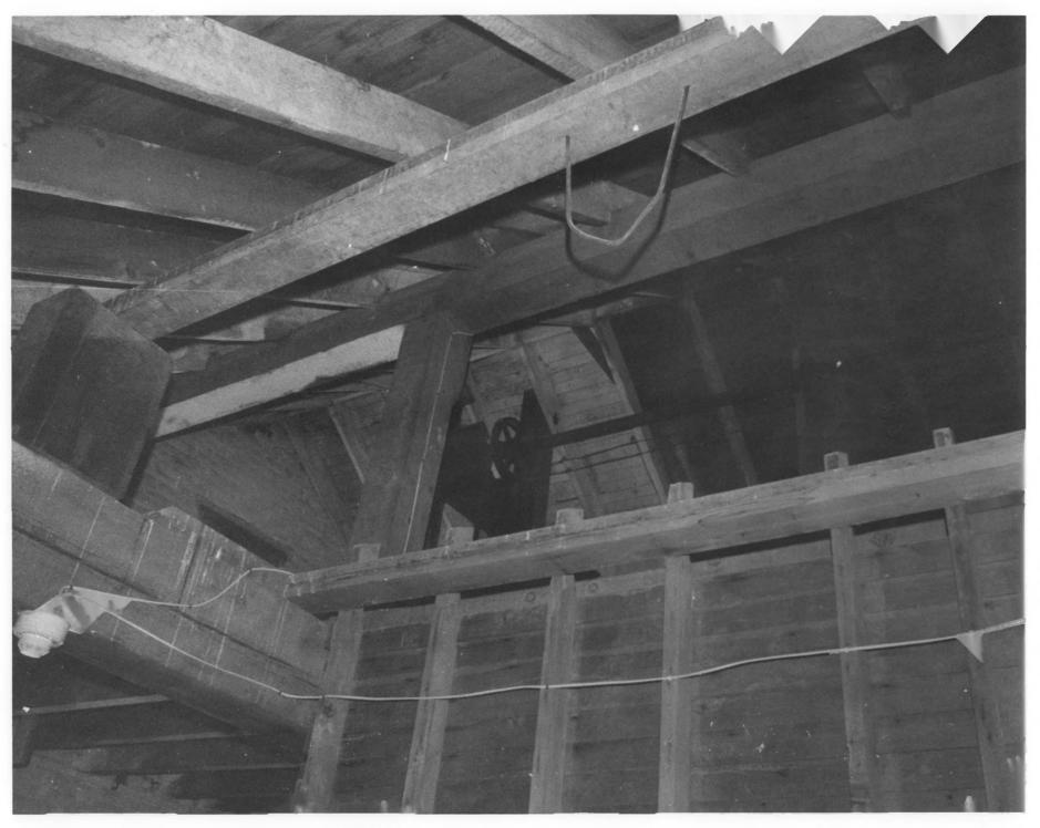
View looking up to roof and loft area from third floor showing massive beams, machinery, and top of one of a number of storage bins within the mill. White object (lower left) is a smoke alarm installed in recent years.
