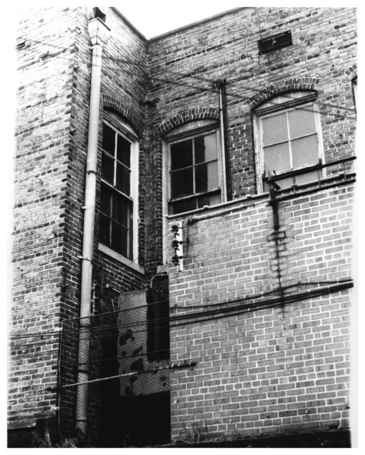
Detail-rear of building-2nd story windows-segmental arch vouissoirs over solid fill lintel. Double hung 4/4 iron frame windows with fireproof glass. Brick 5 rows stretchers between headers
