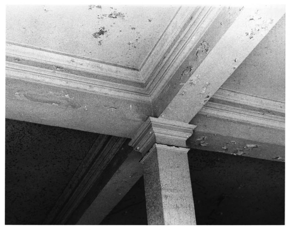
Detail-Interior-concrete ceiling-12"x24" reinforced concrete beams and 24"x24" column
