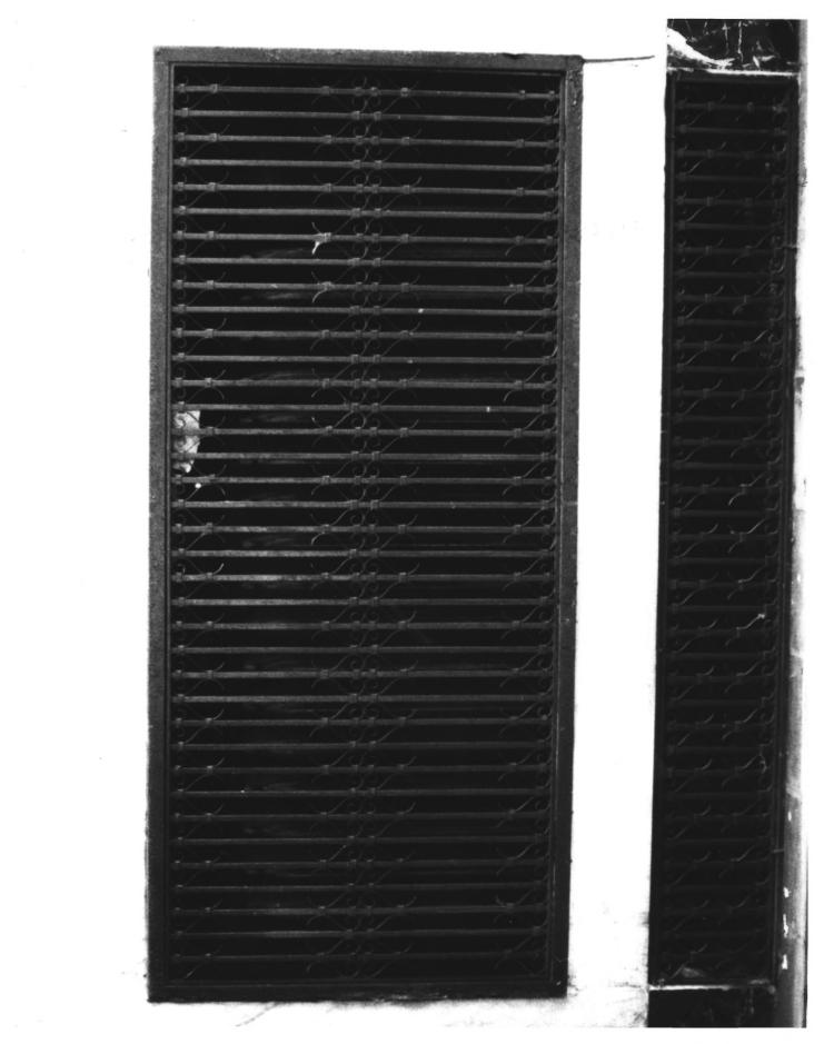
Detail-Interior- Wrought iron grill to heating system in wall #
