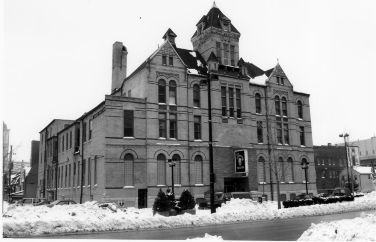
The Milwaukee Turners faces West. Note the glass block windows which cover stained glass windows seen only from the inside. The three stories on the left were added about 10 years after the original construction and are cantilevered to the main building.
