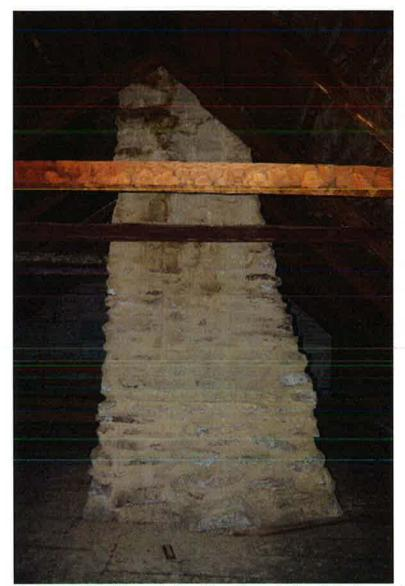
**Photo 25**. Detail of the west side of the chimney in the attic looking east showing significant slope towards the south and front of the house. The visible collar beam is a replacement.
