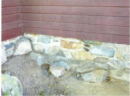
Photo 3 - Cement rich pointing mortar at Southeast corner of North elevation at removed porch
