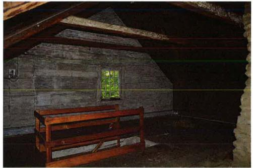
Photo 22. Attic looking southeast to the stairwell and east and south walls showing a corner of the chimney, roof framing, and floor boards. Ghost marks of a nineteenth-century window are visible north of the window, and twentieth-century knee wall cabinets are visible along the south wall.
