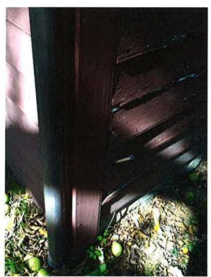
Photo 10 - Probing indicates localized decay; easy knife penetration to 3" depth, SE corner
