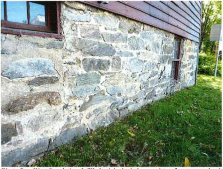
Photo 3a - West foundation. Infilled original window, variety of mortars and pointing techniques
