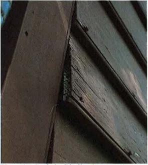
Photo 10a - Typical nail jacking due to cupping
