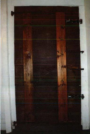
Photo 13. Entrance foyer detail of the interior main entrance door, looking south. The metal strap hinges are visible on the left side of the door frame.
