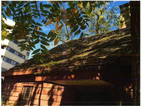
Photo 24 - View of later entry shed and minimal overhang along balance of façade. Note debris accumulation in gutters.
