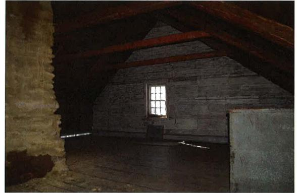
**Photo 24.** Attic looking southwest towards the west attic wall. Ghost marks of a nineteenth-century window are visible north of window, and the two collar beams to the west of the chimney are replacements.
