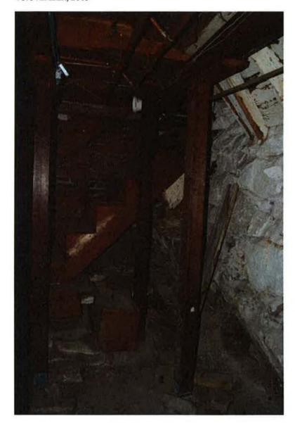
**Photo 26**. Cellar looking east showing wood stairs, showing stone ledge at the east side of the foundation and at the base of the north side of the stone chimney. The bracing for the Keeping Room hearthstone, brick infill wall at the stair, and added support posts are visible.
