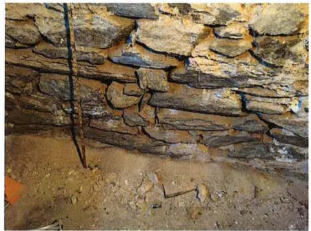
Photo 4 - North wall, basement. Mortar has fallen away from joints. Deposition and texture is not characteristic of having been displaced by water.
