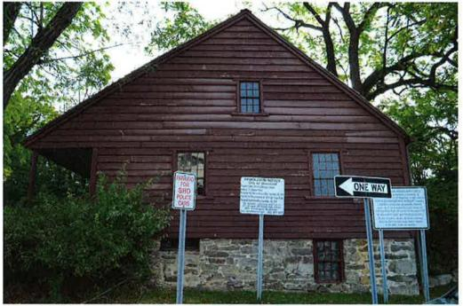
**Photo 6.** West elevation of the Hoyt-Barnum House, looking east from the Bedford Street sidewalk. The ghost marks for the former full-size window at the north side of the foundation are visible.
