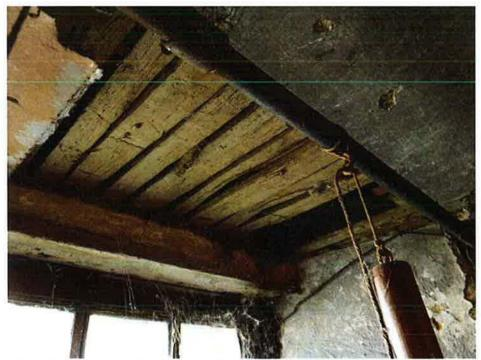
Photo 32 - NW corner, basement ceiling exposed riven lath
