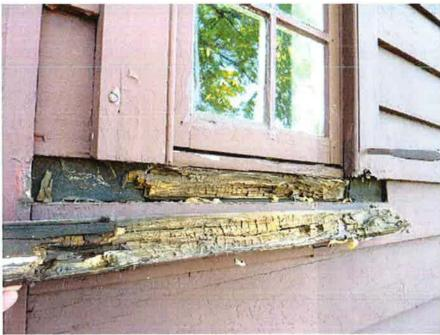
Photo 17a - Toilet window, exterior, rotted sill
