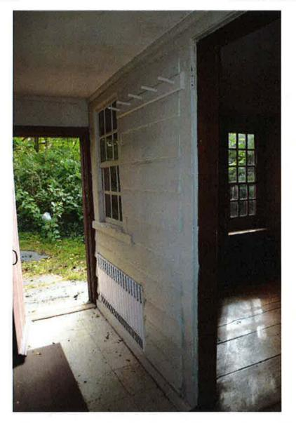
**Photo 21.** Rear ell looking east to the exterior at the east elevation and through an original exterior entrance to the Buttery. The white wall with original clapboards and window was once the original exterior north wall.
