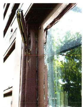
Photo 11 - Rotted jamb, East elevation, SE Room
