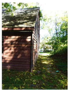
Photo 6 - South Elevation, east side, clapboard in contact with grade.
