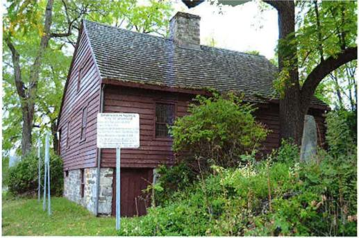
**Photo 5.** South and west elevations with original cellar access door at the west side of the south elevation within the at-grade fieldstone foundation, looking northeast from the Bedford Street sidewalk.
