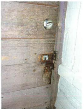
Photo 15d - No surviving interior latch; rim lock replaced by deadbolt
