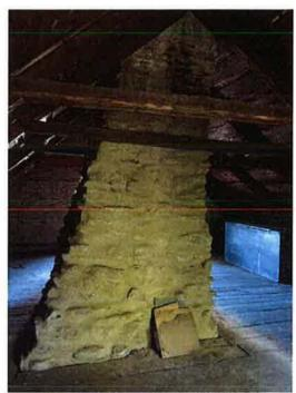
Photo 31 - Chimney cant through attic. Note mortar-wash stain at upper extent.
