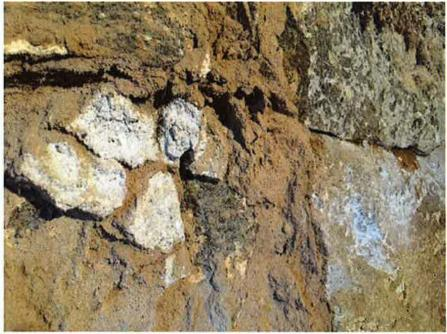
Photo 5 - Mortar displacement consistent with insect activity.
