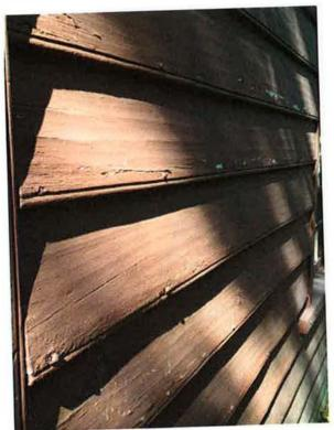
Photo 8 - Detail of clapboard
