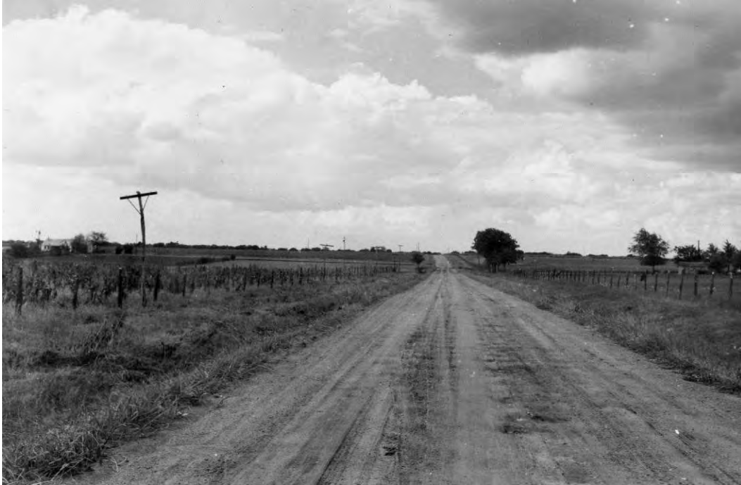
Figure 38. FM 155 in Fayette County before improvement. (Source: TxDOT Library)
