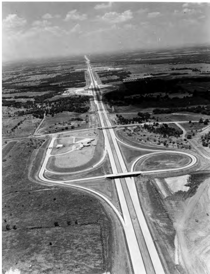
Figure 46. Dallas-Fort Worth Turnpike (now IH 30) interchange at Watson Road (now SH 360), 1957. (Source: www.texasfreeway.com .)
