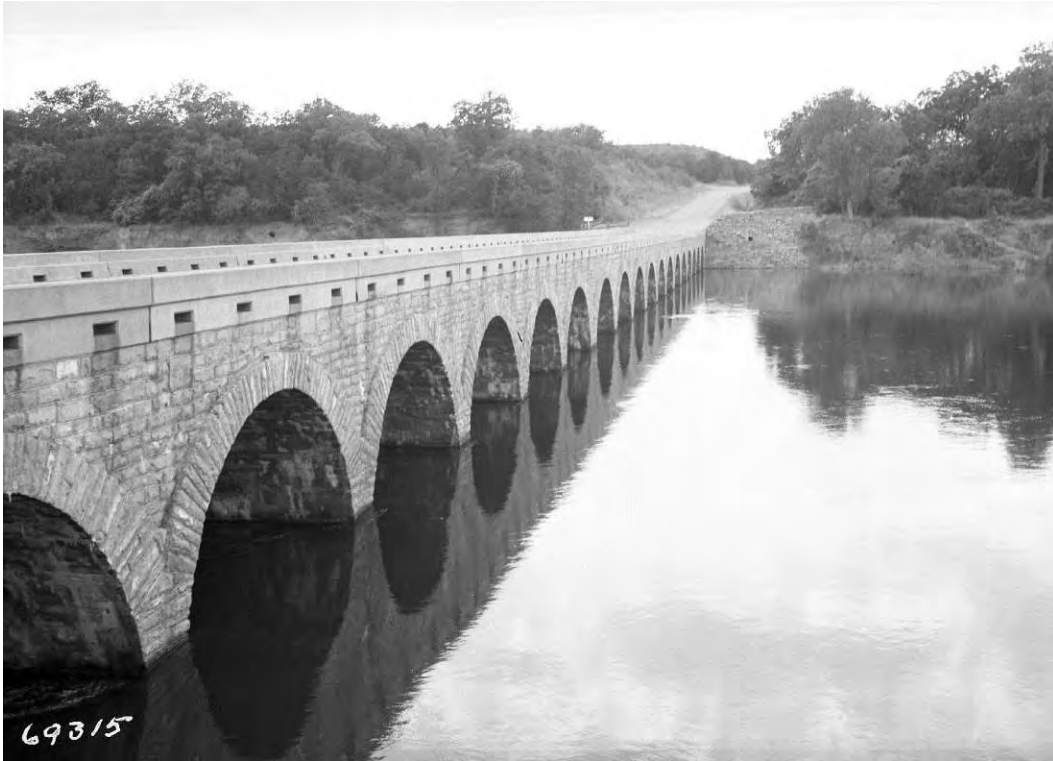
Figure 30. Possum Kingdom Bridge at the Brazos River, early 1940s. (Source: Texas Department of Transportation Photo Library)
