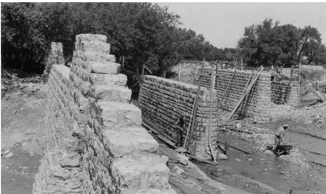
Figure 29. Use of stone masonry on THD project in Erath County, late 1930s. (Source: Texas Department of Transportation Photo Library)
