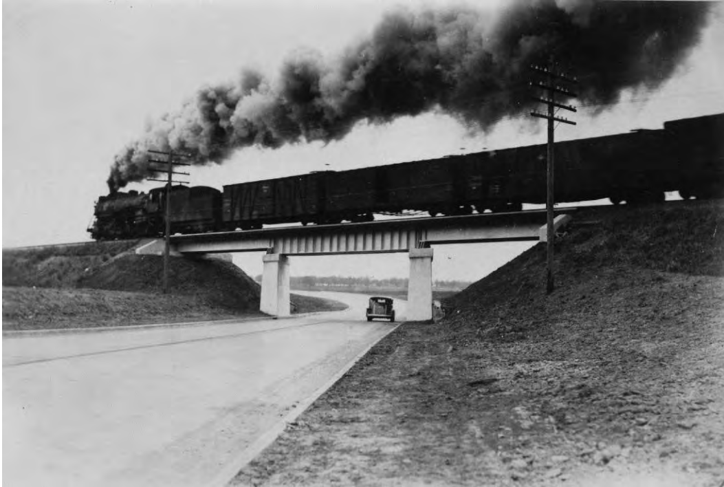
Figure 37. Recently completed grade separation structure, US 81 in Montague County, November 1936. (Source: Texas Department of Transportation Photo Library)
