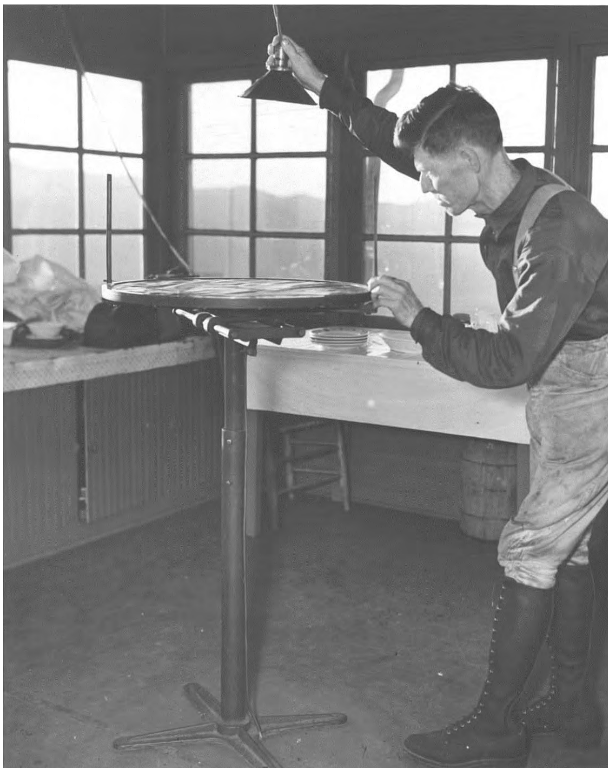
Figure 3. A TDF ranger demonstrating use of the alidade in a fire lookout tower on Hemlock Mountain, ca. 1938. Photo courtesy of the Tennessee State Library and Archives.
