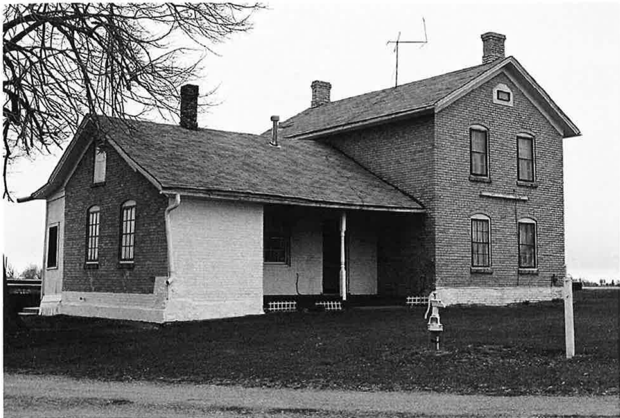
Figure 8. Another view of the Wolter Farmhouse with the formal two-story wing on the right. This house is one of about three Chaska brick farmhouses in Carver County that retain a shed-roofed porch tucked into the massing. Note the brick walls on three sides of the porch, and the single wooden column supporting the edge of the roof. Wolter Farmhouse, Co. Rd. 33, Young America Twp., Carver Co. (facing NE, photo by Barbara J. Henning, 2004).
