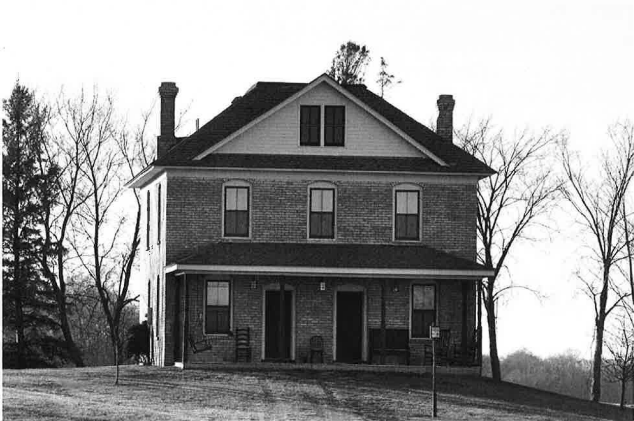
Figure 12. About 10% of Carver County's Chaska brick farmhouses have hipped roofs and boxlike massing. This example in south central Carver County was built ca. 1900. Note the flanking brick chimneys. Two entrances on the main facade is an unusual feature found in some German immigrant communities nationwide and rare in Carver County. Farmhouse, Co. Rd. 51, Benton Twp., Carver Co. (facing W, photo by Scott Kelly, 2011).
