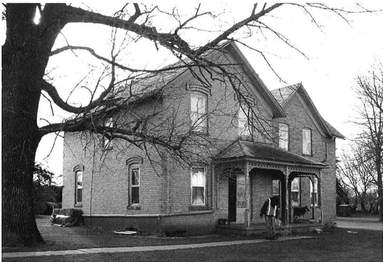
Figure 10. Another view of the Hesse Farmhouse. Ornamentation on most Chaska brick farmhouses is confined to the brickwork above the segmental-arched windows and wooden detailing on porches. Windows on the eastern half of the Hess Farmhouse (at left in the photo) have projecting brick hoods. Those on the western half have a double row of flush brick headers forming the arch. Hesse Farmhouse, built ca. 1885, Co. Rd. 41, Dahlgren Twp., Carver Co. (facing SW, photo by Scott Kelly, 2008).
