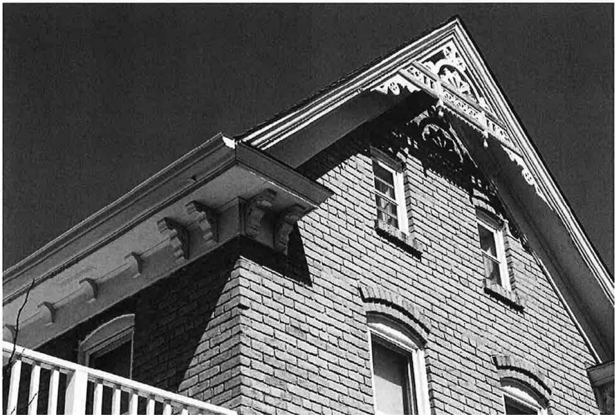
Figure 14. While most of Carver County's brick farmhouses are somewhat austere, some have wooden detailing in the gable ends and at the eaves. This is the Buschkowsky Farmhouse, built in 1894 in northeastern Carver County. (The nearby Heck Farmhouse – listed in the National Register – is about the same age and has a similar form and detailing.) Buschkowsky Farmhouse, Audubon Road, Chanhassen Twp. (now City of Chanhassen), Carver Co. (facing NE, photo by Barbara J. Henning, 2004).
