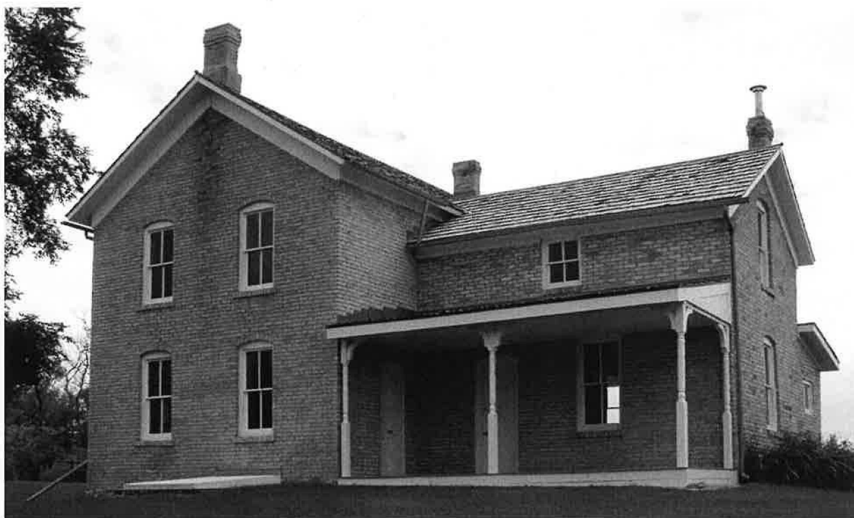
Figure 4. This Chaska brick farmhouse, built in 1876, is a T-shaped example of the cross-wing form with a shed-roofed porch at the intersection of the wings. The western facade (around the corner at the left end of the photo) has two widely-spaced windows on the first story, two windows directly above them on the upper story, and no entrance. The house is typical in its sparse ornamentation. Recently restored, the property was listed in the National Register for its associations with the original owner, German immigrant Wendelin Grimm, who settled in Carver County in 1857 and developed a hardy strain of alfalfa that helped transform Midwestern dairying. Wendelin Grimm Farmhouse, Grimm Road, Laketown Twp., Carver Co. (facing N, photo by Todd Murray, August 2009).
