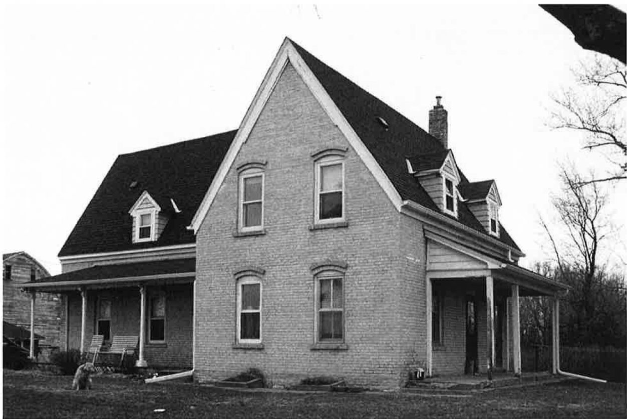
Figure 11. This farmhouse, built in two phases in 1891 and 1894, has a cross-wing form and a roof pitch that is unusually steep. The small dormers are rare among Carver County's brick farmhouses. Each wing of the house is about 15' x 30'. The southern facade (at left) faces the road while the more formal eastern facade (at right) faces away from the farmyard and outbuildings. The original owners were Bavarian immigrants Mathias and Maria Jacobs who established the farm in the late 1850s. The farm was 136 acres in the 1890s when the house was built. Jacobs Farmhouse, Hwy. 212, Dahlgren Twp., Carver Co. (facing NW, photo by Scott Kelly, 2008).
