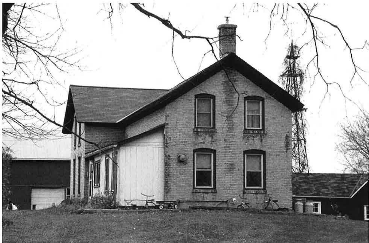
Figure 5. An L-shaped Chaska brick farmhouse in southeastern Carver County. The house was built in two phases in 1873 and 1883 with wings measuring about 16' x 26' and 17' x 28'. The main facade, which faces the road, is on the left in the photo. The house has a typical alteration: enclosure of the front porch. Frank Farmhouse, Hwy. 212, Dahlgren Twp., Carver Co. (facing W, photo by Scott Kelly, 2008).
