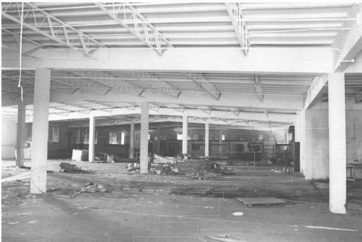
Fig. 15: Interior view of a factory in Cidra: shows concrete columns and beams, steel joist and precast concrete roof slab panels. Photo: Guillermo Marrero, 2012
