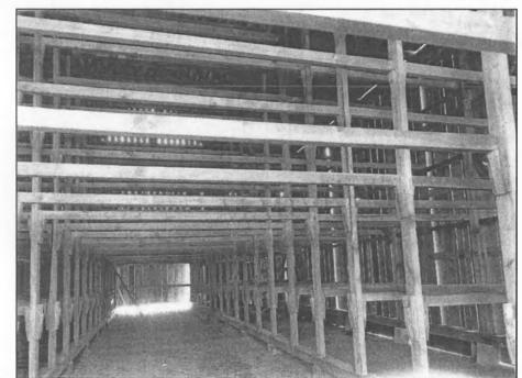
Figure 9. Interior view of the framing system of a single-aisle tobacco barn Records of the Maryland Agricultural Experiment Station 1929
