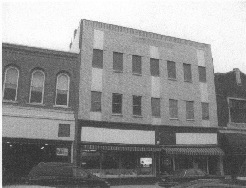
Figure 45: Bookin Building with post-1947 façade (2007 photos)
