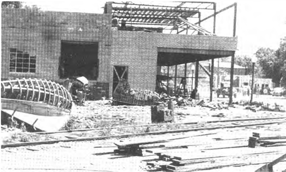
Figure 49: Yates Building under construction, 1947 flood (Disaster at Ottumwa, Iowa)
