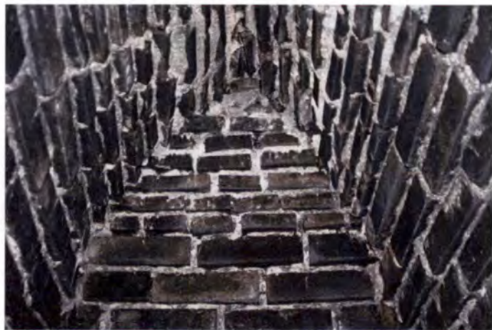
Figure 4: March 28, 2008 Interior of Fejeran hotno showing layered firebricks and afok to the top.
