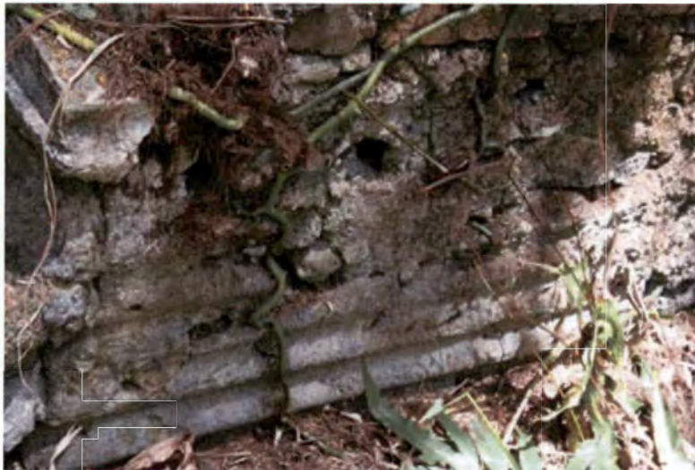
Figure 5: The pattern of corrugated tin is seen in the base of the Sugiyama/Paulino hotno at Acho Lasodiac property.
