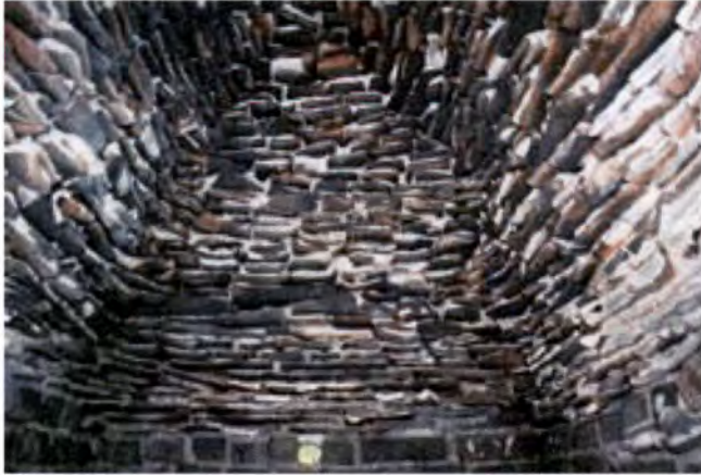
Figure 6: Interior of Sugiyama/ Paulino hotno showing the exhaust hole at the bottom center to the roof.
