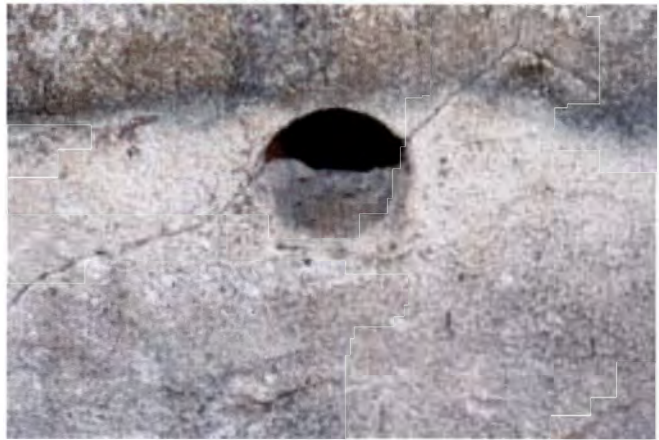
Figure 5: March 28, 2008 This photo of the Fejeran's hotno shows the hole built into hotnos to regulate heat inside.
