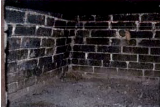
Figure 3: March 4, 2008 Inside view of Jose Cruz Fejeran hotno showing the ladriyu and afok layers of the hotno's construction.
