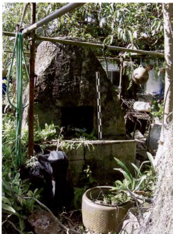
Photo 13. Cruz Oven, Barrigada. The camera is facing southeast. The photo stick is one meter long. Note that the oven base is constructed of cement hollow blocks.
