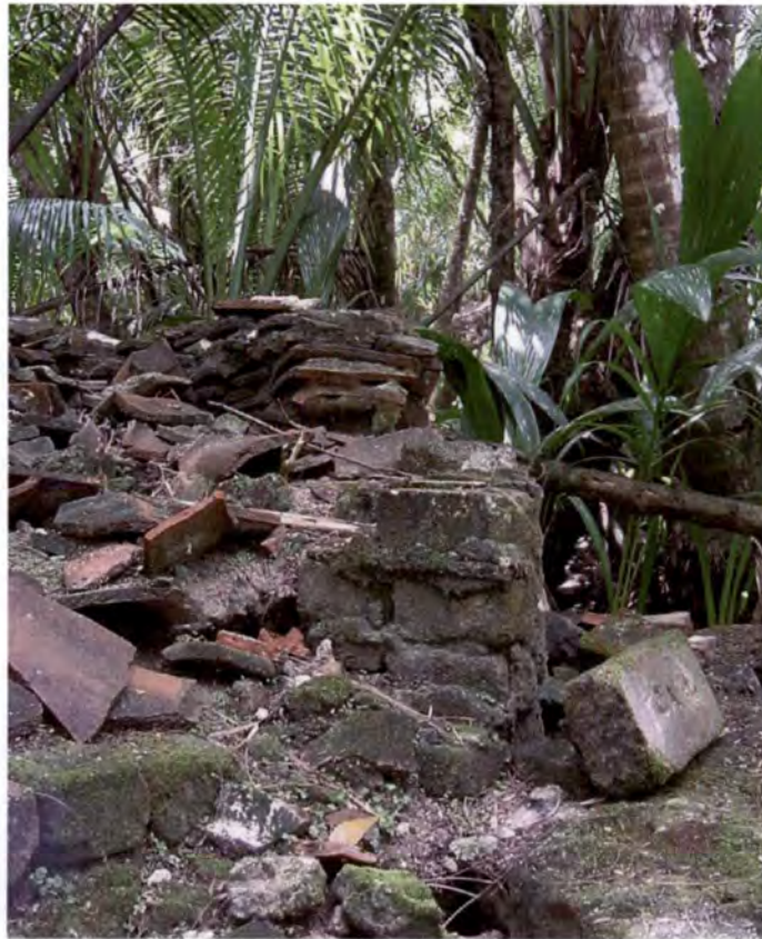
Photo 5. Close up of the right side of the Sella Bay Oven vault showing the brick and tile construction techniques. The camera is facing southeast.
