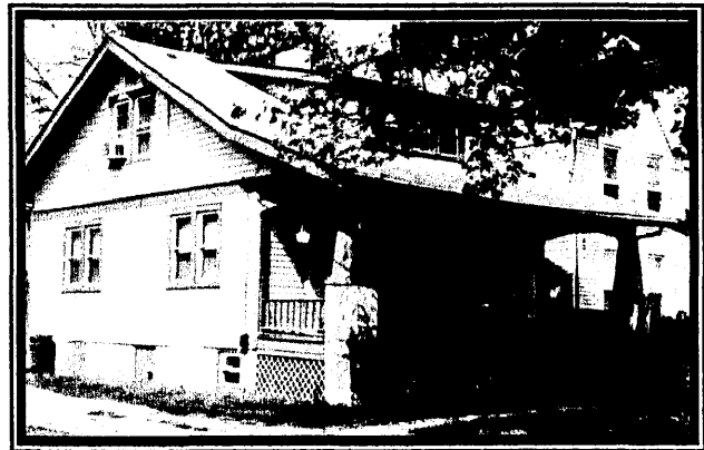
Much of the character of Erlanger's residential areas is defined by twentieth-century design, including Bungalows such as this 1½-story home, with a recessed front porch and dormer.
