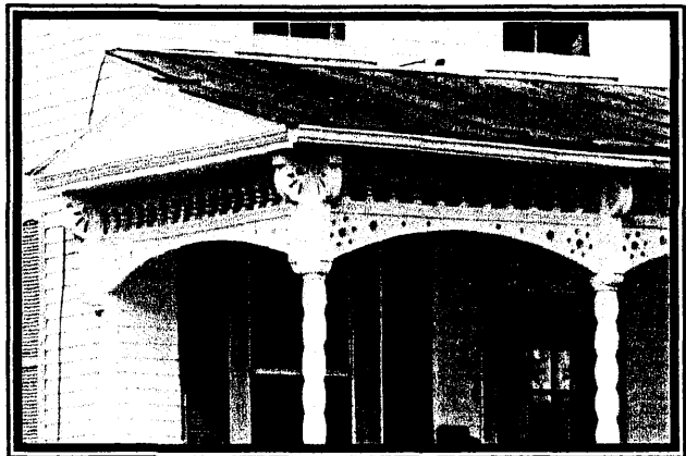
Some of Erlanger's late nineteenth-century homes, such as this handsome property at 3214 Crescent Avenue, retain their distinctive Eastlake-style porches, incorporating lathe-turned posts and balustrades.
