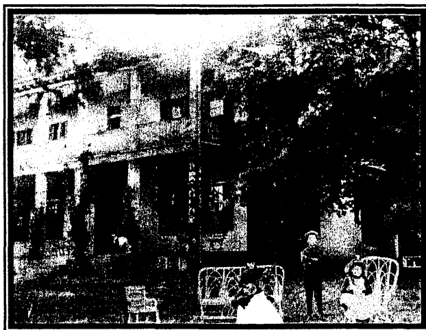
"Walnut Grove," the Bartlett Graves House, built in the 1820s (destroyed)
