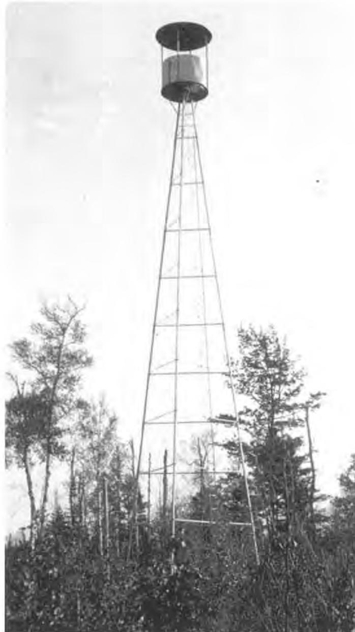
Figure F3. Some of Minnesota's earliest steel towers, like the unidentified example shown here, had three rather than four legs. The first cabs on steel towers were cylindrical, enclosing the open crow's nest. No examples of three-legged towers or towers with open platforms or cylindrical cabs have survived. Minnesota Historical Society collection.
