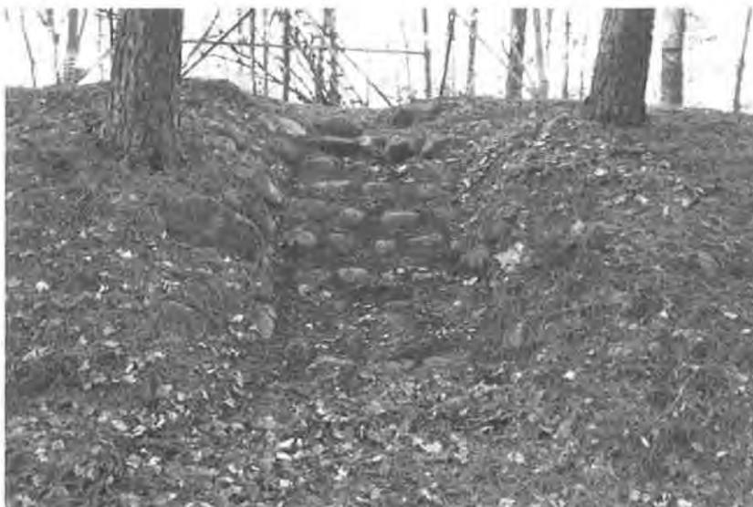
Figure F21. Rare CCC-built stone steps leading to the Ben Draper Tower. The flanking hillside is riprappd with stones. 2014 photo by Gemini Research.
