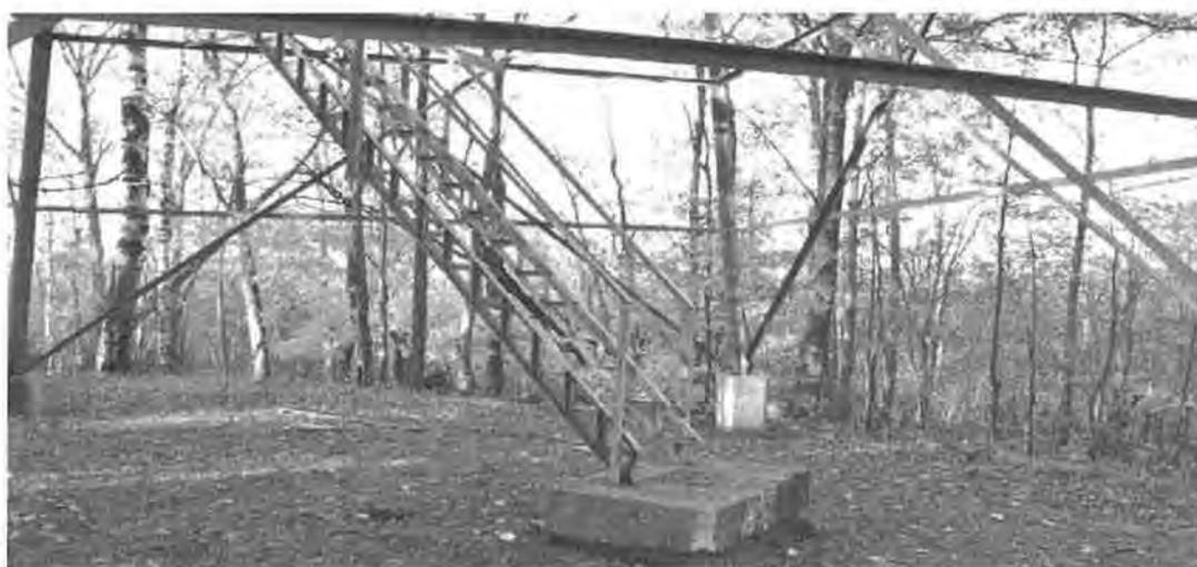
Figure F16. The stairs and their concrete footing at the Ben Draper Tower. The tower was erected by the CCC for the Minnesota Forestry Division in Land O'Lakes State Forest, which was established in 1933. It is a 100' tower fabricated by Aermotor. The 42" by 48" footing is signed and dated by the CCC. The tower is 24' square at the base and its largest members are 5" steel angles. 2014 photo by Gemini Research.
