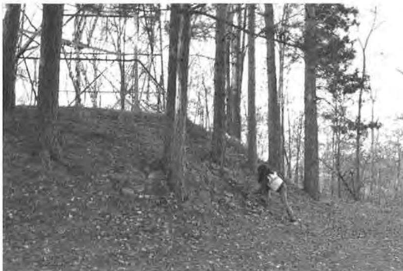
Figure F20. The CCC improved many Minnesota lookout tower sites. Some towers, like the Ben Draper Tower (1937) shown here, are still surrounded by CCC-planted pines. The CCC also protected the summit of this tower by placing stone riprap (mostly obscured by leaves) on the steep slope. Extant examples of this type of site element are rare. 2014 photo by Gemini Research.
