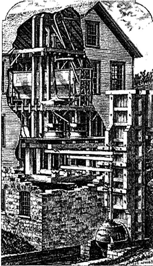
Fig. 3 Superior efficiency, all-season usefulness, and low cost led the American mixed-flow type turbine (which channeled water inward and then downward) to displace the traditional overshot wheel and others. Illustrated here is the method of transmitting power from the turbine to run two millstones. ("Leffel Turbine Wheel Driving a Two-Run Flouring Mill," *United States Miller*, 16(January 1884), 37)
