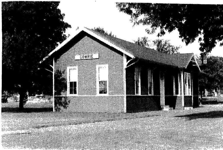
Plate 6: Rock Island Depot at Gowrie, 1899 restored and moved to city park
