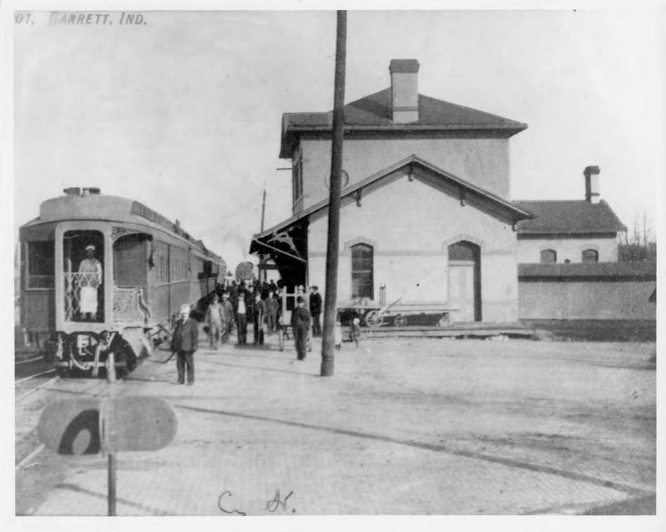
Photo 7. View of the West elevation of the passenger depot prior to 1910 remodelling, which added a full second story to the building
