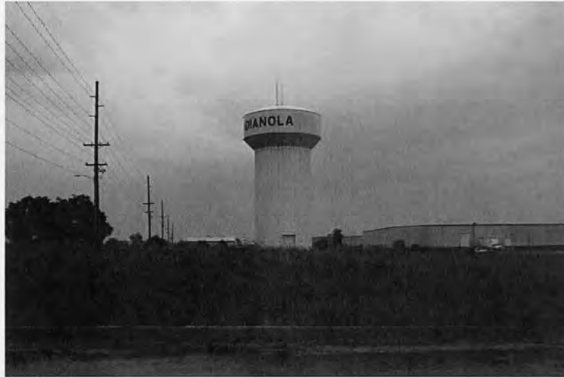
Figure 13. WATER TOWER TYPOLOGIES – HYDROPILLAR
