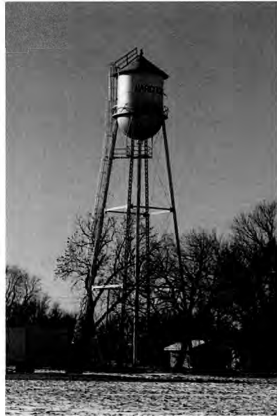
Figure 8. WATER TOWER TYPOLOGIES – HEMISPHERICAL BOTTOM (Riveted or Welded)
