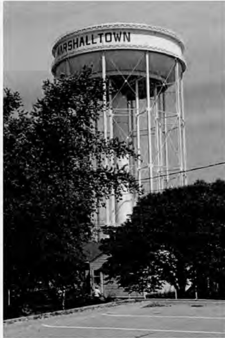
Figure 10. WATER TOWER TYPOLOGIES – SPHEROID (TOROSPHERICAL)
