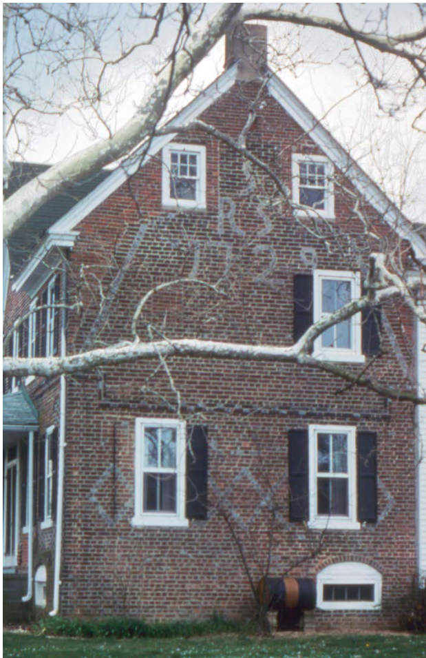
Figure 4 Vitrified brick shows profile of gambrel roof before enlargement to two full stories.
