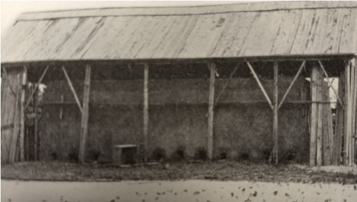
Figure 7 Scove kiln (evolution of the "arches"-type clamp), in NJ, ca.1900
