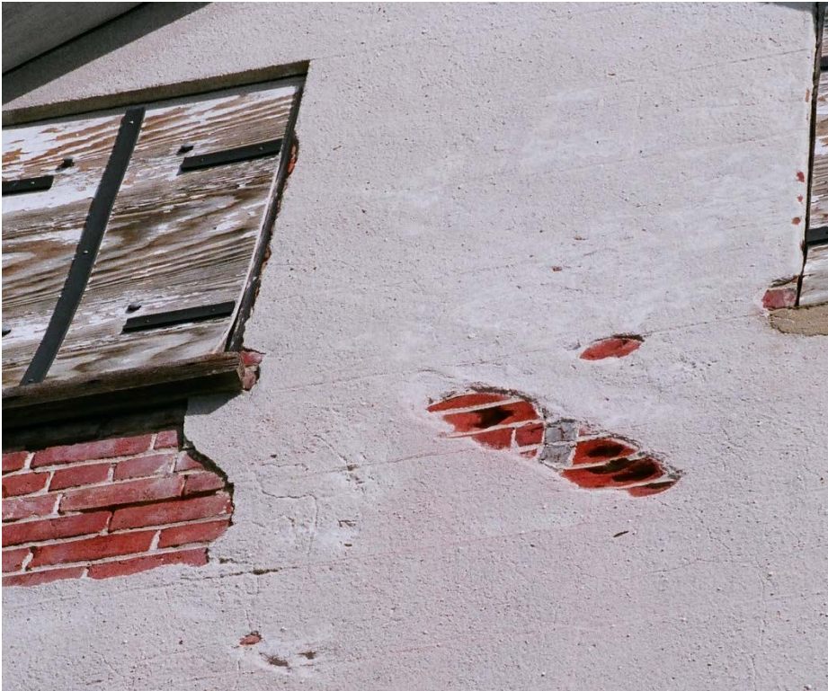
Figure 38 Stucco spalling, slowly revealing a date.
