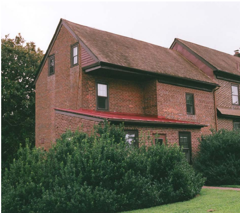
Figure 6 A rare house type, view of rear elevation. This example has a façade of Flemish checker.
