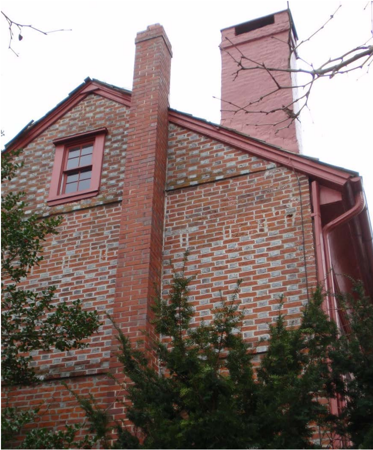
Figure 9 Patterned brickwork comes in both formal versions (above) and vernacular ones.
