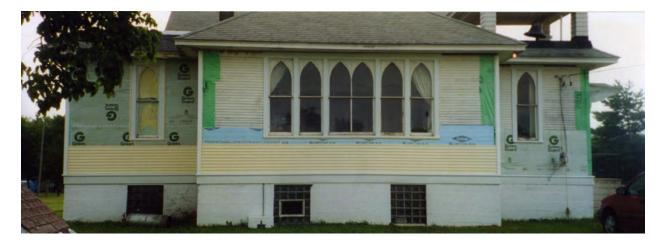
Figure #10 – Work on the siding and roof in 2002, showing both the old wood siding and new vinyl siding. Property of the Littleton and Chatham Historical Society.
