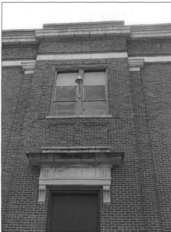
Figure 2: End-entry pavilion, view east (photo by J. Jacobsen, May 6, 2008)
