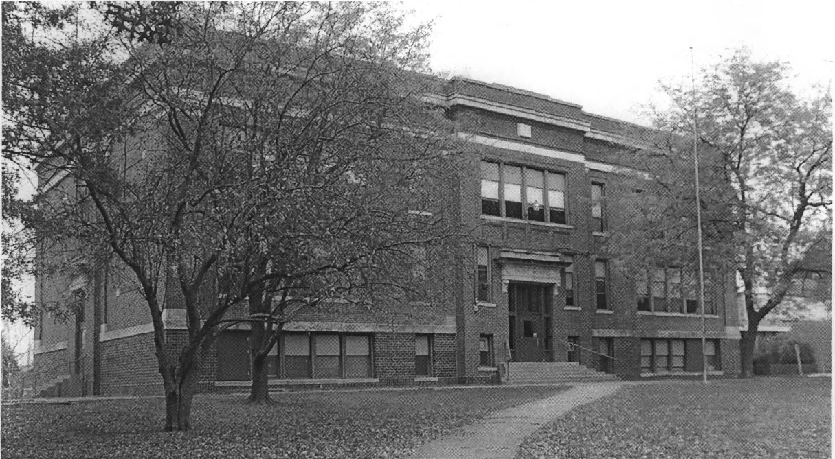
Figure 1: South façade, view northeast (photo by J. Jacobsen, May 6, 2008)
