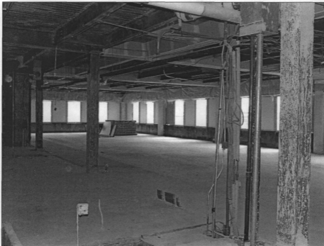
Figure 16: Fourth floor, overview looking southeast (photo by James Jacobsen, August 9, 2007)
