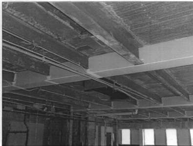
Figure 24: Fourth floor, overview looking southeast (photo by James Jacobsen, August 9, 2007)
