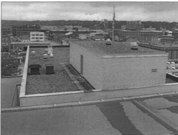
Figure 25: Fourth floor, overview looking southeast (photo by James Jacobsen, August 9, 2007)
