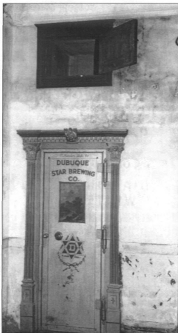
Figure 14: Company safe, ground floor of office area, views west (photo by J. Jacobsen, August 2006)
