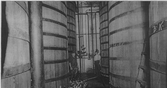
Figure 41: Dubuque Star Brewery, fermenting vats in Stock House, view north, c.1909, note the baskets of wood filter chips just removed from the vats (courtesy of Catherine Collins, Dubuque)
