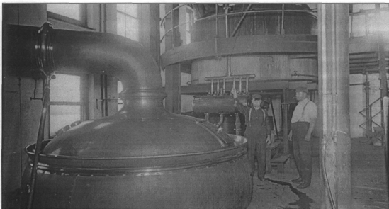
Figure 45: Dubuque Star Brewery, brew kettle and mash tub, grant, second floor of brew house, view south, c.1909 (courtesy of Catherine Collins, Dubuque)
