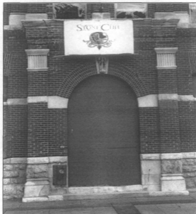
Figure 3: Main entry detail, view west (Photo by J. Jacobsen, August 2006)
