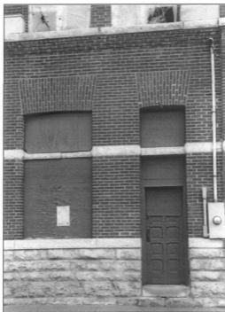
Figure 2: Detail, massive brick arches with vertical coursing on lower openings, view west (Photo by J. Jacobsen, August 2006)
