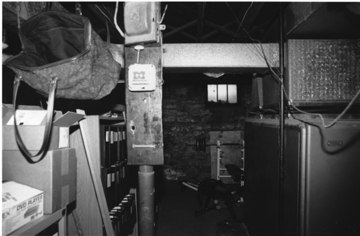
CRAIG - BEASLEY HOUSE WILLIAMSON COUNTY, TN
