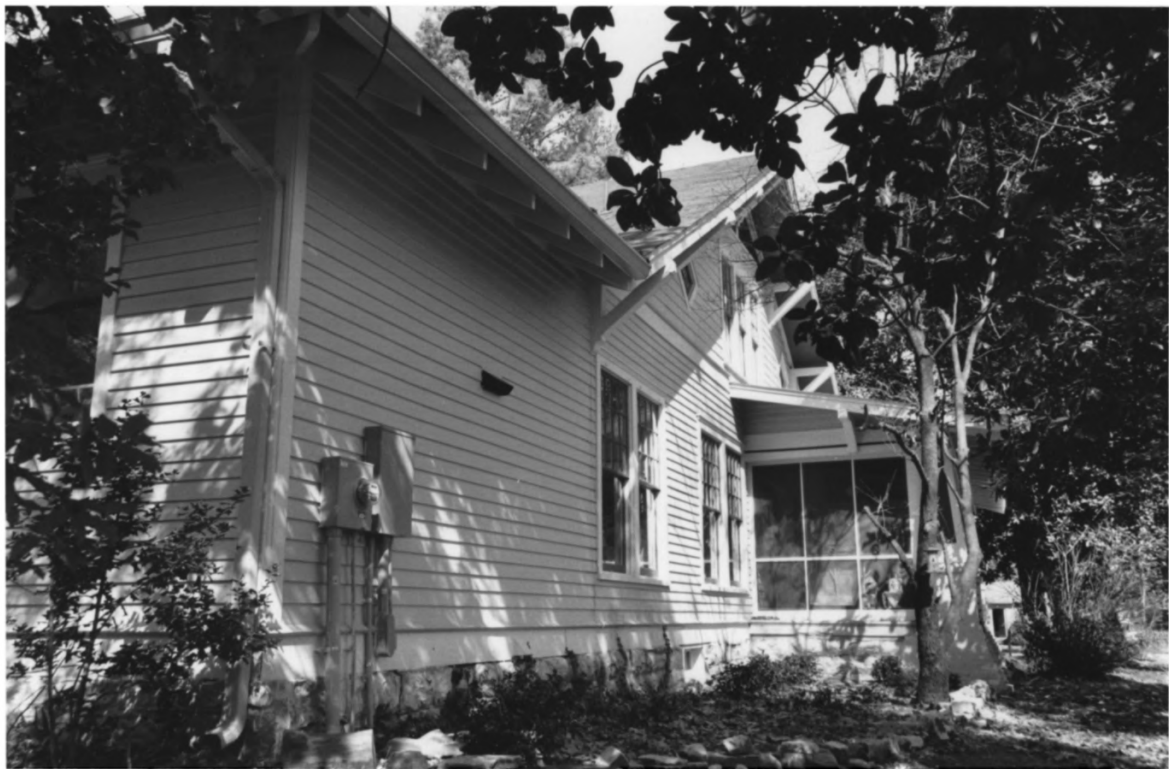
CRAIG - BEASLEY HOUSE WILLIAMSON COUNTY, TN
