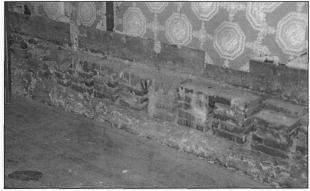
Figure 14: Dropped floor level, back of plan (note baseboard marks) (view northwest, photo by Jim Jacobsen, April 23, 2001)
