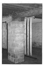
Figure 41: Stone pier (view southeast, photo by Jim Jacobsen, April 23, 2001) (Refer to basement floor plan, shown above)
