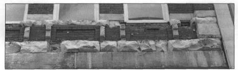
Figure 3: Transom, main floor sill level detail, damage to stonework due to the metal covering (the damage is being repaired) (view west, photo by Jim Jacobsen, April 23, 2001)
