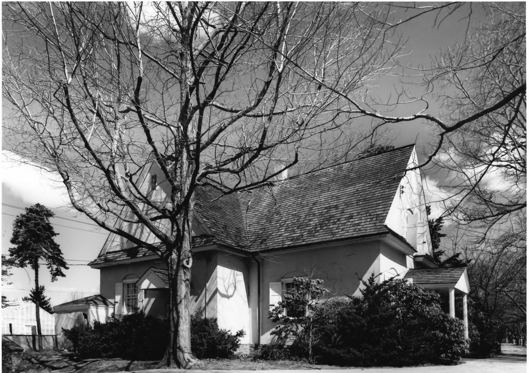
Photo #2 Merion Friends Meeting House Montgomery County, Pennsylvania South and west elevations Anthony S. Bley, 1987
