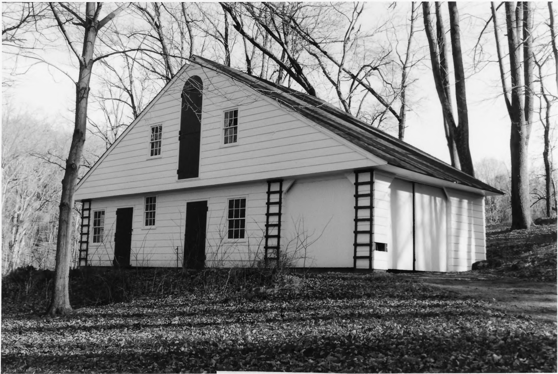
N. C. WYETH HOUSE AND STUDIO Chadds Ford, Pennsylvania Barn facing southeast Photo: R. Wise, 1997
