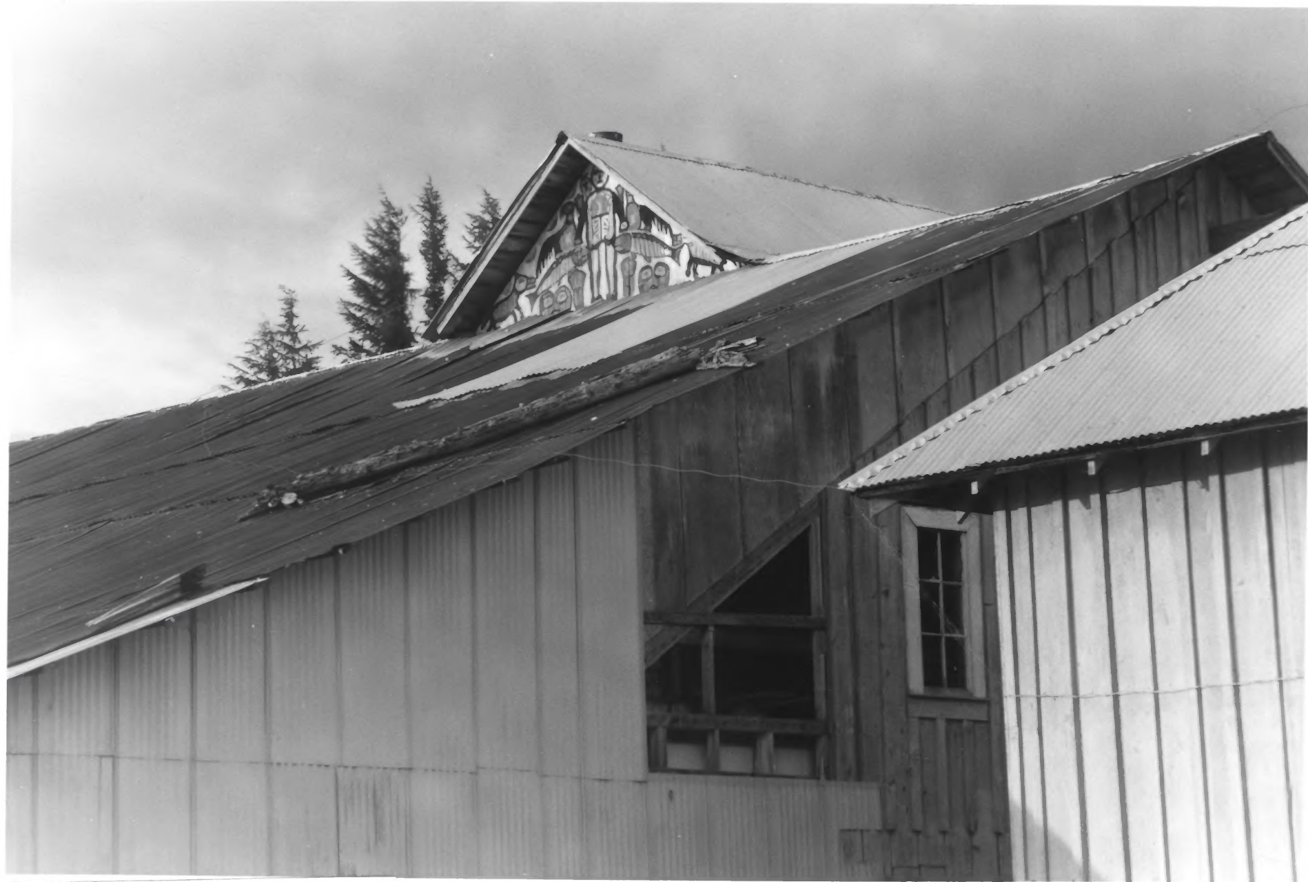
KAKE CANNERY, Kake, Alaska Detail of Mural in Main Cannery Building Linda Cook, 1992
