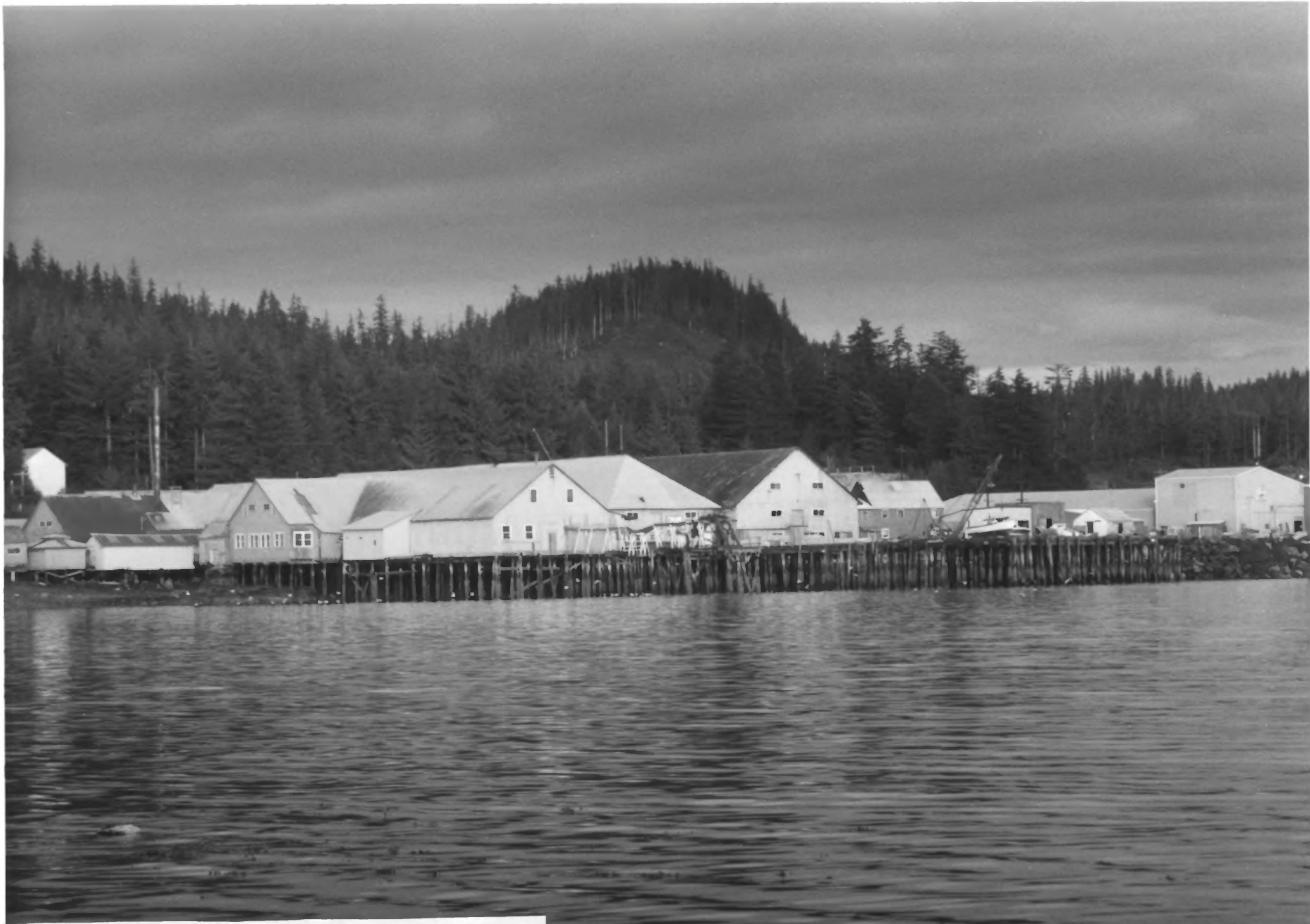
KAKE CANNERY, Kake, Alaska General View of Cannery Buildings from Water
