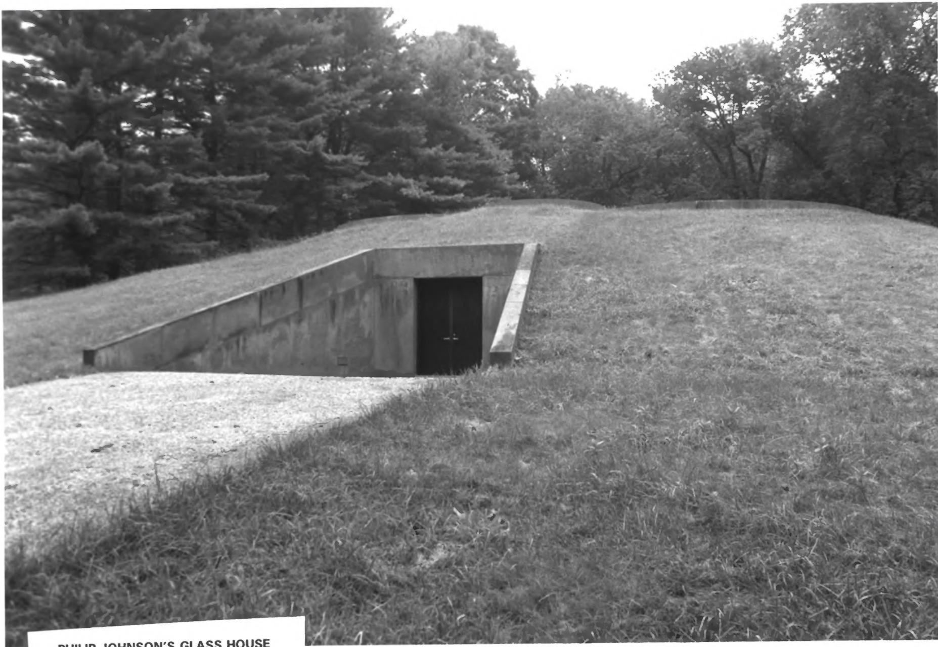
PHILIP JOHNSON'S GLASS HOUSE Fairfield County, Connecticut Painting Gallery Photo: Historic Resources Consultants, Inc., July 1996
