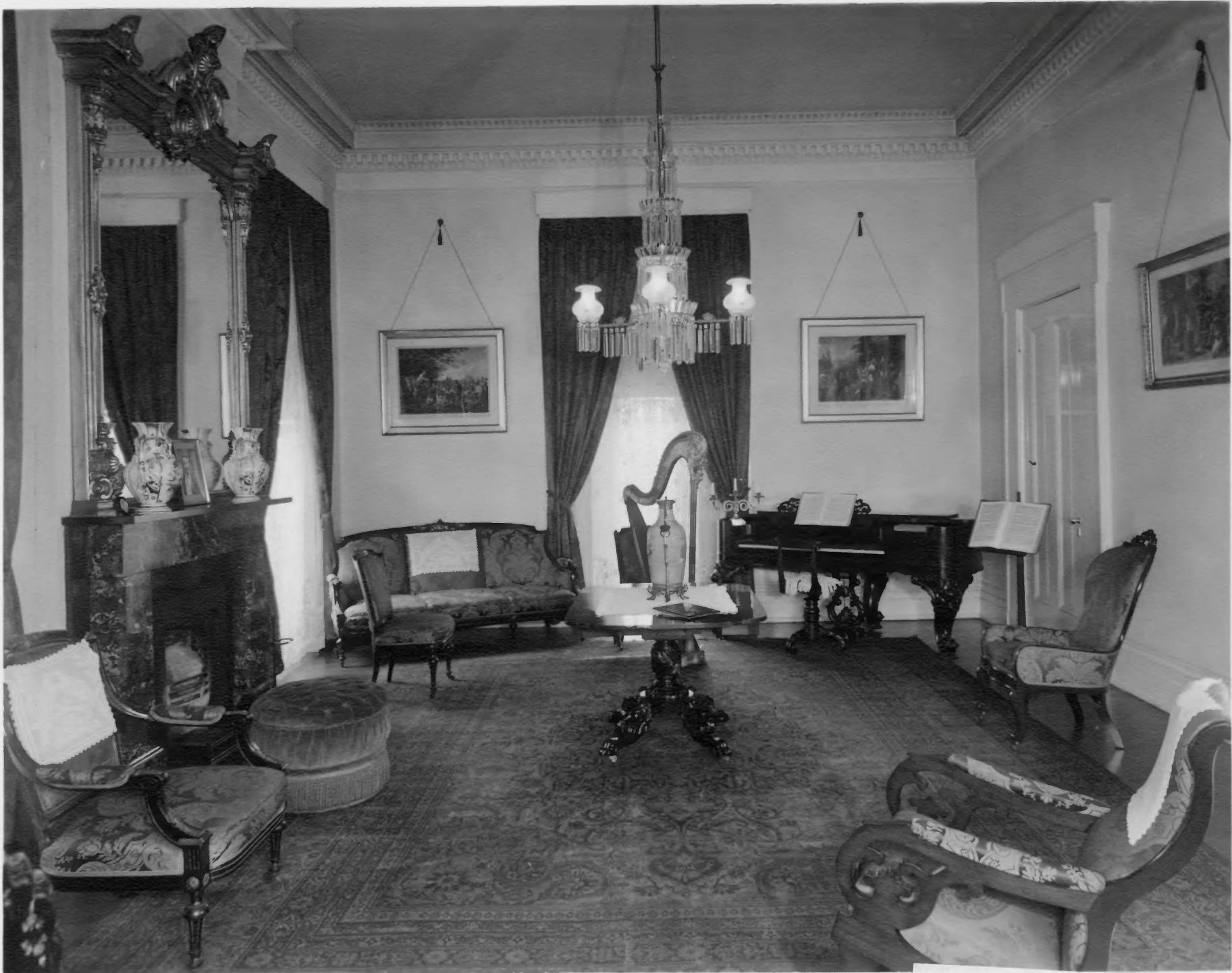
Lanier Mansion Madison, Indiana North Double Parlor Photo: Indiana SHPO
