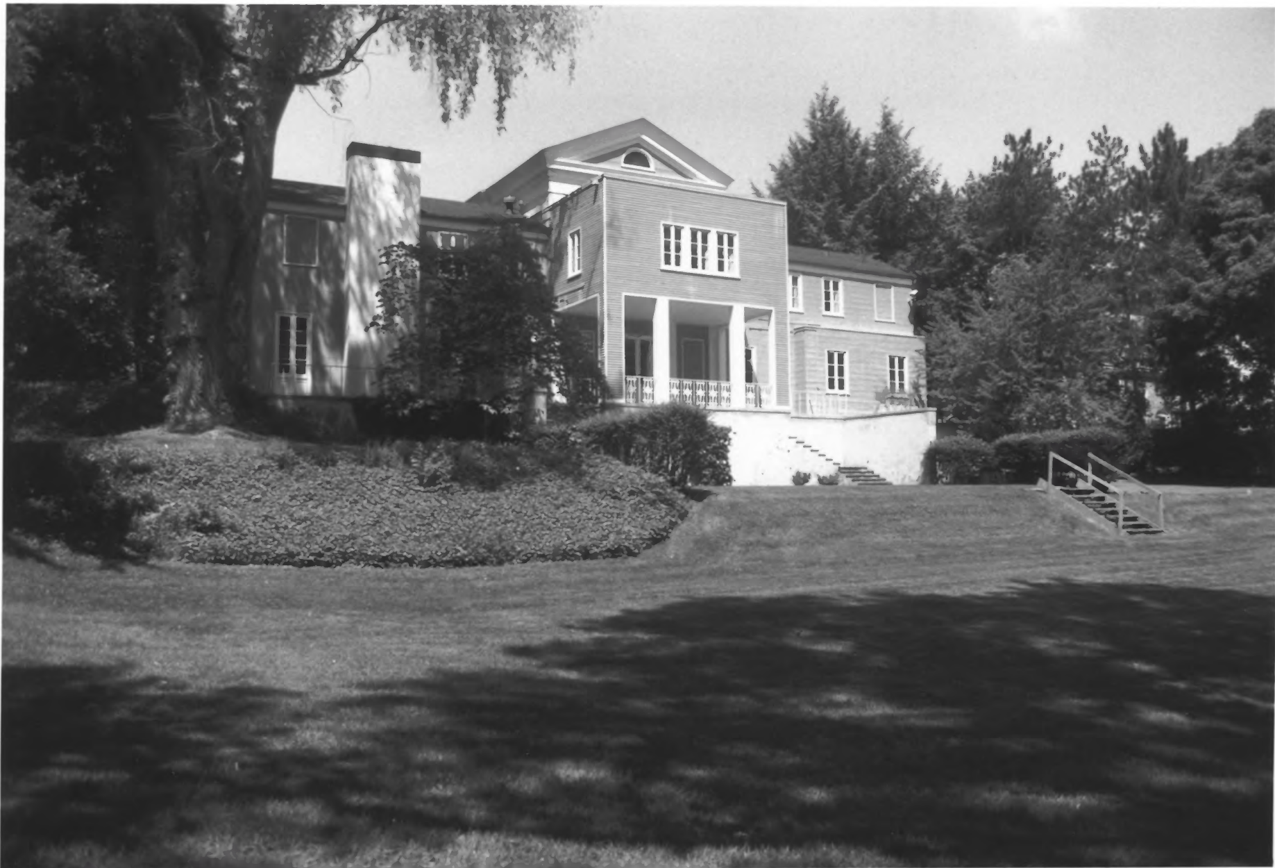
The Austin House Hartford, Connecticut Rear elevations, view northwest Photo: David Ransom, 1993
