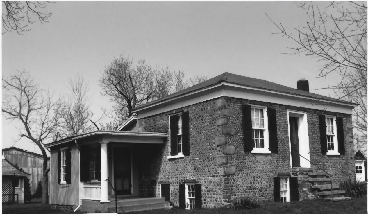
Cobblestone H.D. Childs, NY Ward House (Parsonage) Front & West Elevation Photo: Nancy Todd NY SHPO, 1992
