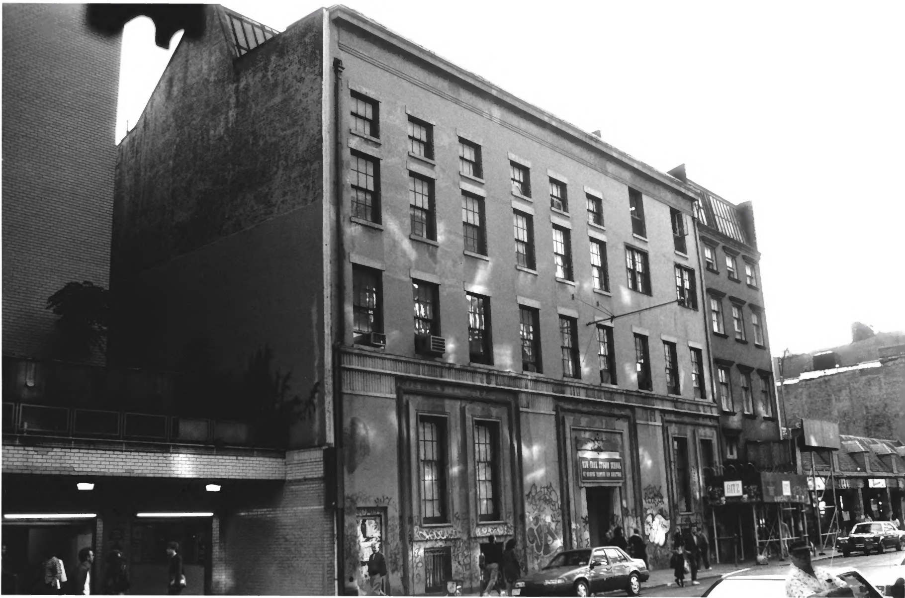
WHITNEY MUSEUM OF AMERICAN ART New York, New York Front Facade facing on West 8th Street Photo by Douglas Morgan, October 1991
