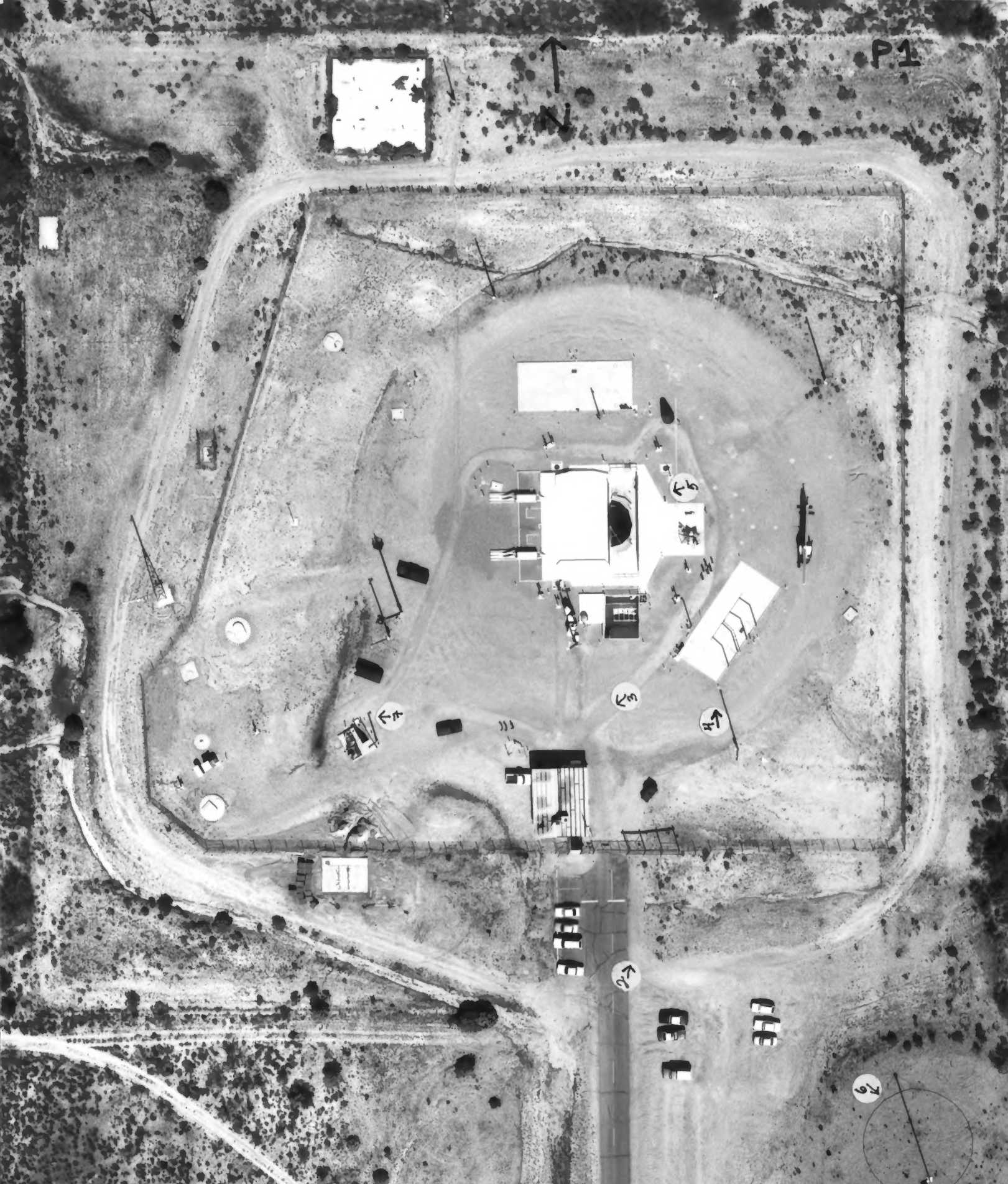
Photograph #1 Titan II ICBM Missile Site 8 (571-7) Green Valley, Pima Co., Arizona Aerial view during conversion of site to a museum. (Angles of photographs #2 - #7 are indicated) Cooper Aerial Survey, Tucson, AZ, 1987
