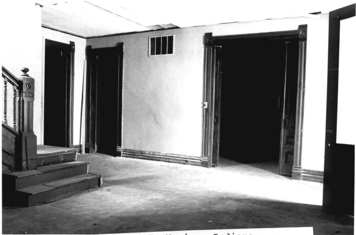
MARIE WEBSTER HOUSE, Marion, Indiana Craig Leonard, Bufton, Indiana, October 1991. Facing northwest, from front parlor of house.
