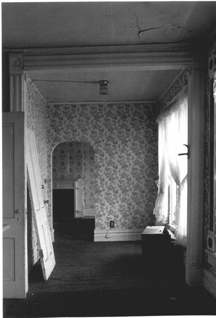
MARIE WEBSTER HOUSE, Marion, Indiana Craig Leonard, Bufton, Indiana, October 1991 Rooms on east side of the 2nd floor.
