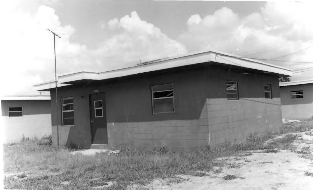
ZORA NEALE HURSTON HOUSE Fort Pierce, Florida Southeast corner of house and south front Photo by Hal Kelly, August 1989
