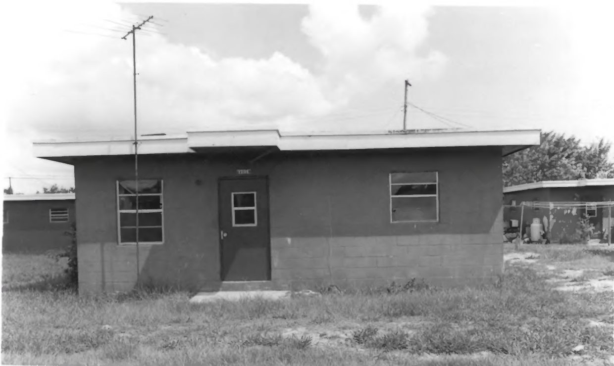
ZORA NEALE HURSTON HOUSE Fort Pierce, Florida South side of house showing front door Photo by Hal Kelly, August 1989
