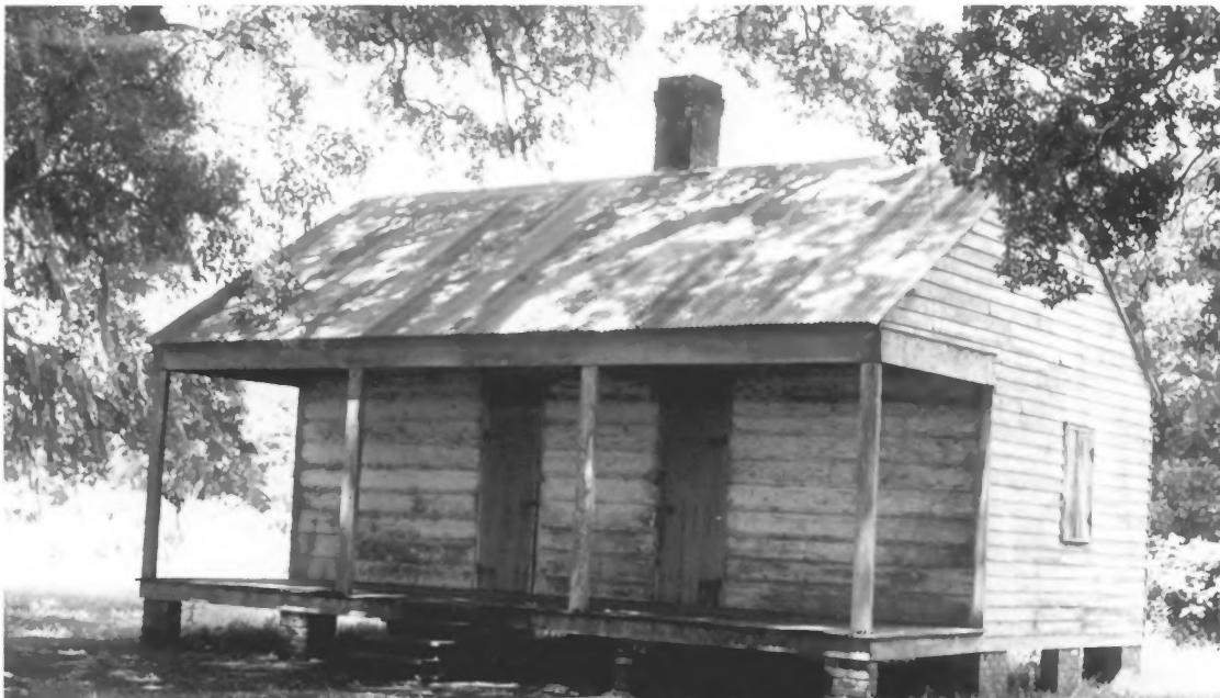
EVERGREEN PLANTATION St. John the Baptist Parish, Louisiana Two room slave cabin Photo by Donna Fricker, May 1991
