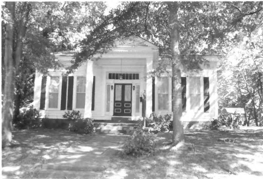
4) Fish Pond House, Corinth Battlefield Corinth, Mississippi Front Facade, view looking east Paul Hawke, Photographer; September 26, 1990
