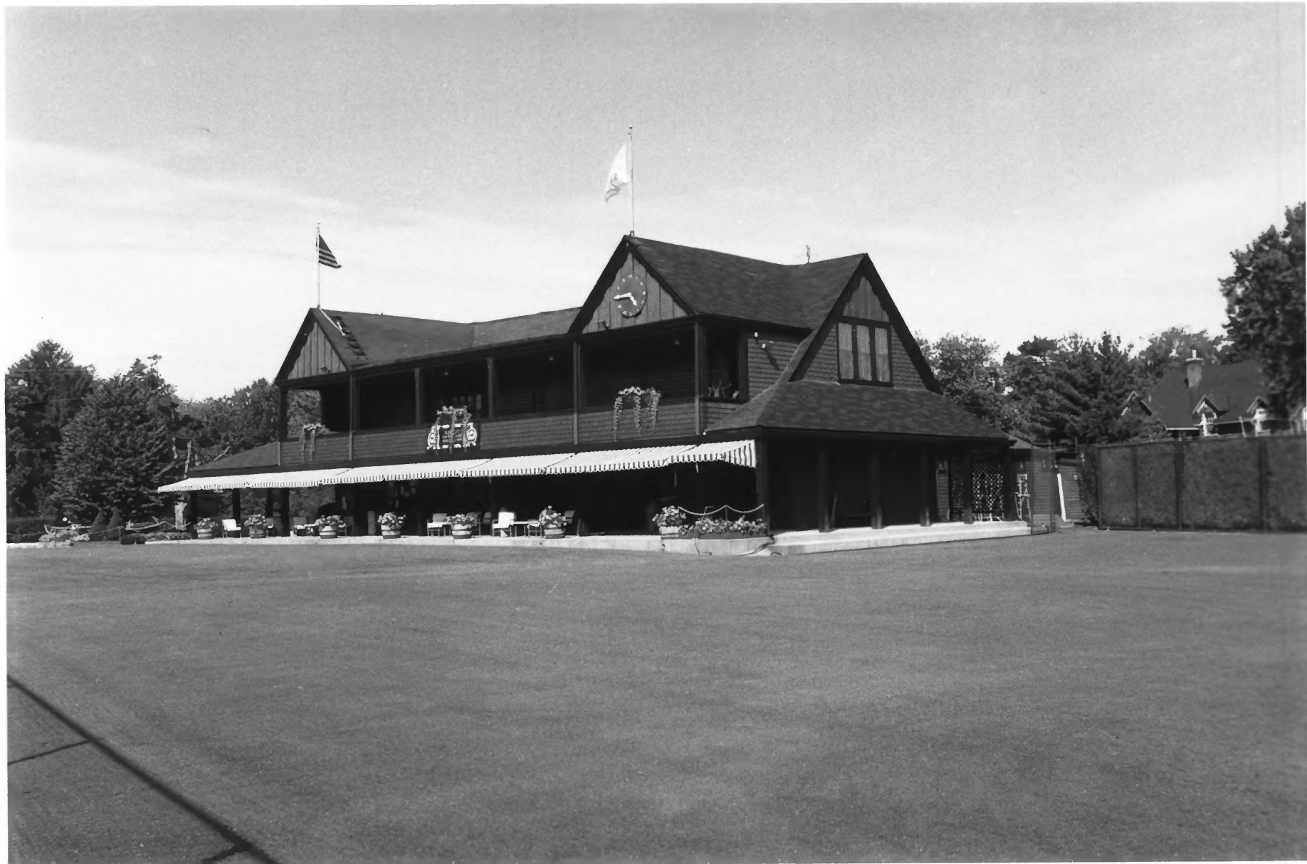
Seabright Lawn Tennis and Cricket Club, Rumson, N.J. Photo 2: clubhouse, south (front) and east elevations (Constance M. Greiff, PHOTO 2 of 10 1990)
