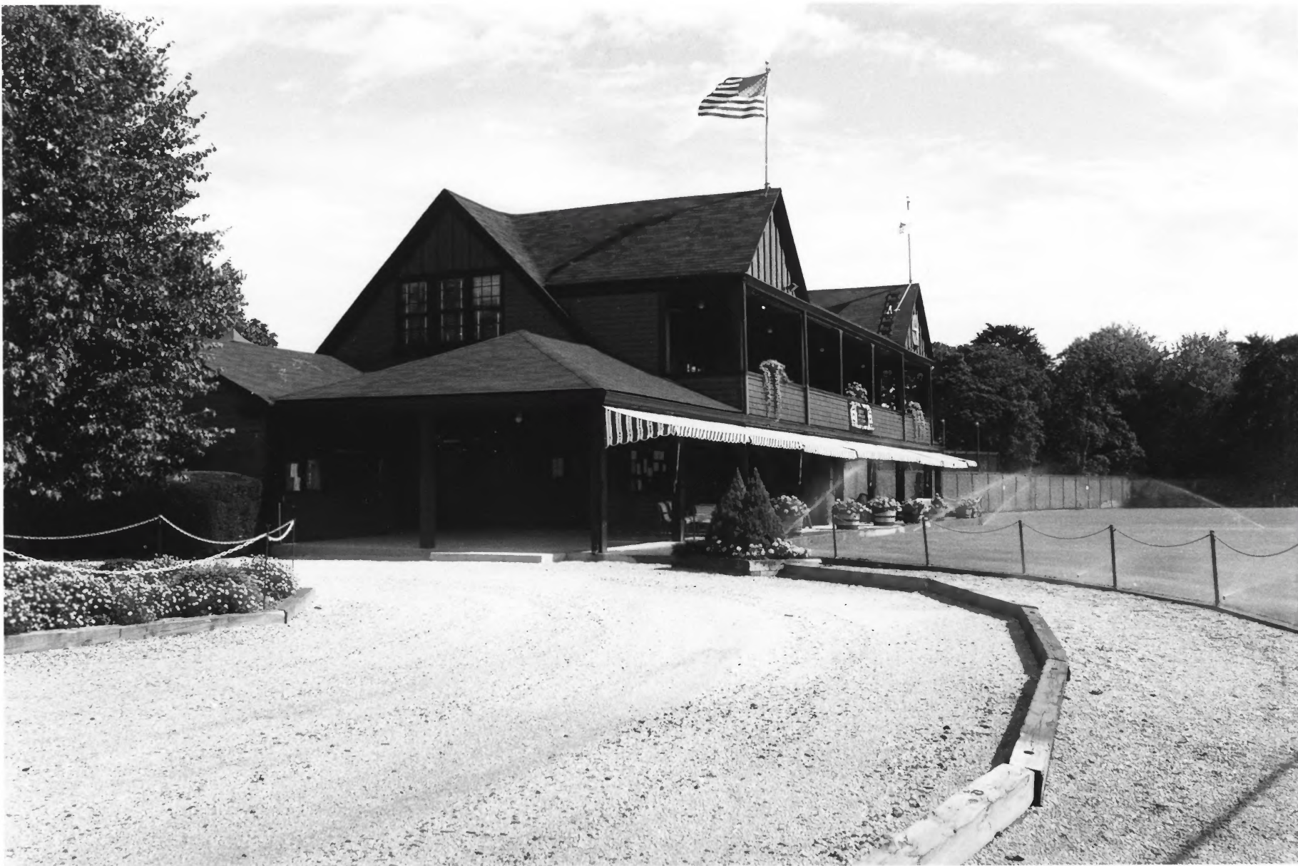
Seabright Lawn Tennis and Cricket Club, Rumson, N.J. Photo 3: clubhouse, south and west elevations (Constance M. Greiff, 1990)
