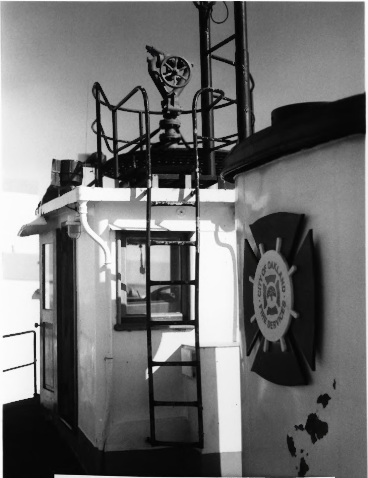
FIREBOAT CITY OF OAKLAND, EX-HOGA OAKLAND, CALIFORNIA Owner: UNITED STATES NAVY BOAT DECK, SHOWING PILOTHOUSE, STACK, AND ORIGINAL PILOTHOUSE MONITOR. Photo #5 by JAMES P. DELGADO, 1988 Courtesy of: NATIONAL PARK SERVICE
