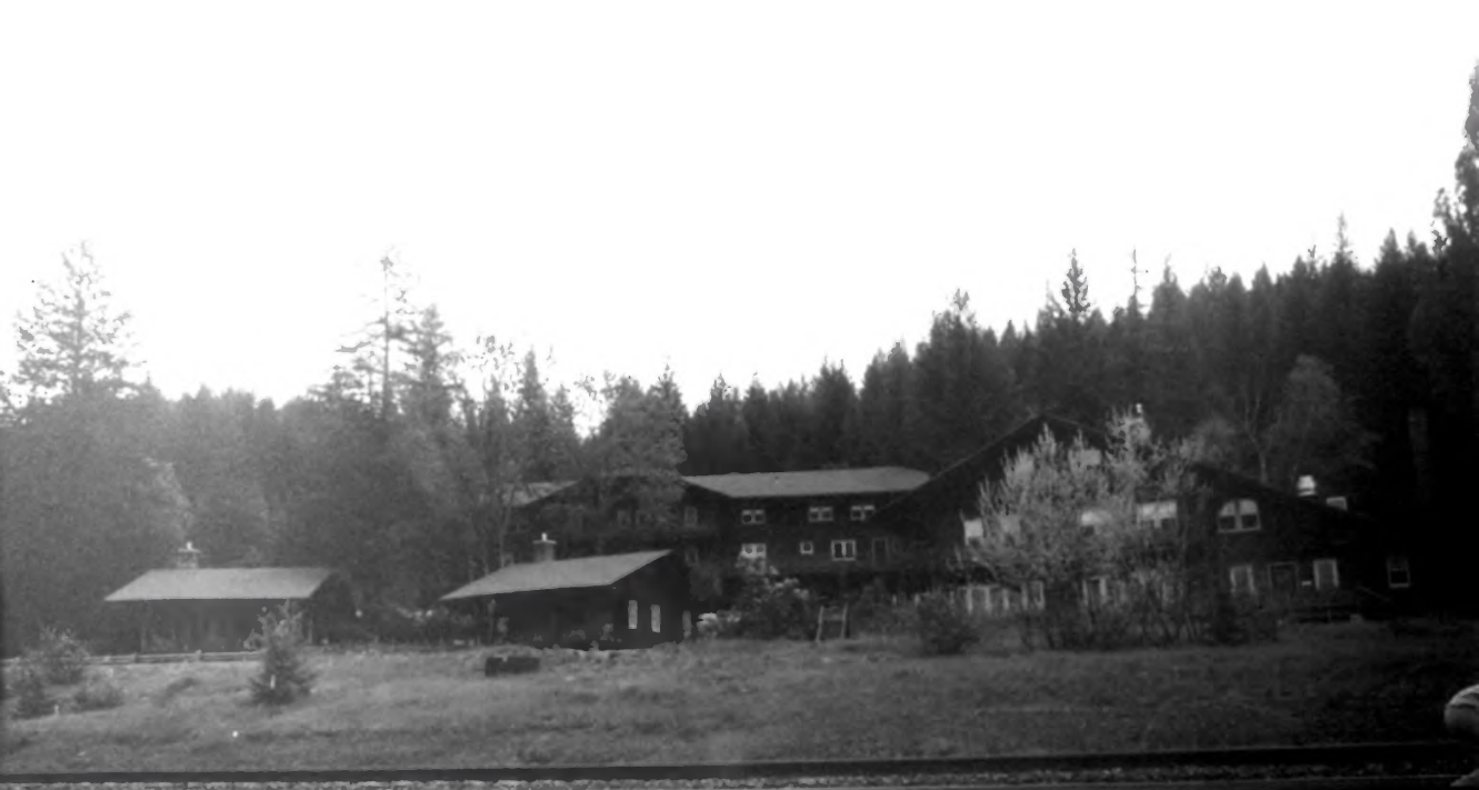
Figure 1 Great Northern Railway Buildings (Boundary Increase) Flathead County, Montana Overview of Belton Chalet Complex, from the railroad tracks Photographer: Ann Emmons May 1999
