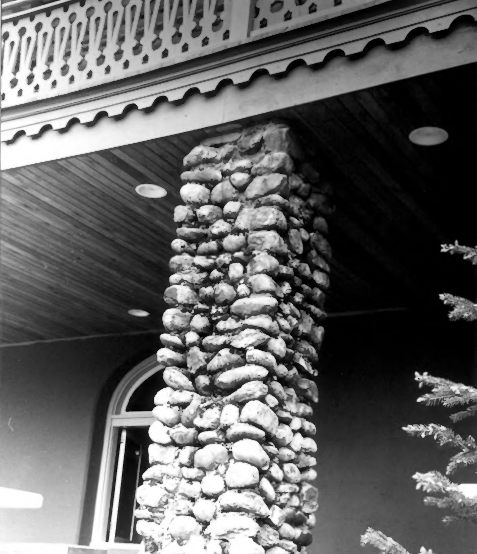
Figure 11 Great Northern Railway Buildings (Boundary Increase) Flathead County, Montana Column detail, dormitory Photographer: Ann Emmons May 1999
