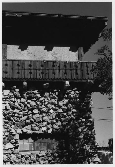
Southeast corner of Grand Canyon Power House showing details of stone and concrete work and balcony railing detail.
