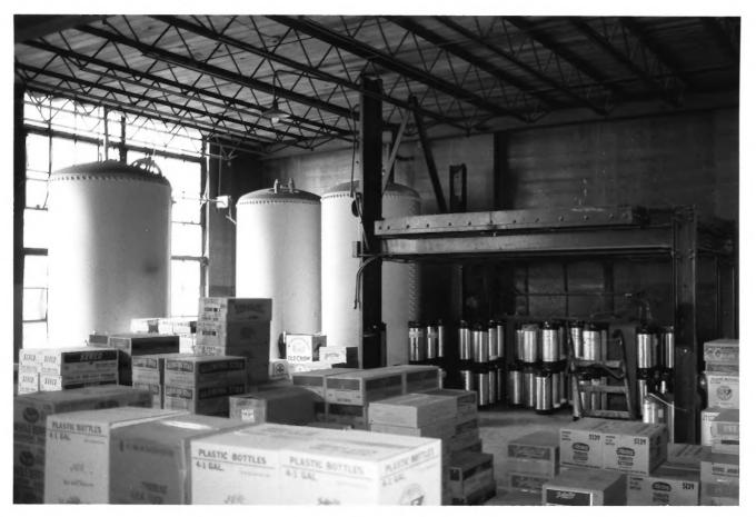
Grand Canvon Power House interior. Tanks and heavy steel work on the right are original. Space framing and wood decking above are recent additions, but are totally removable and are not attached to the structure. Grand Canyon National Park NPS photo by Laura Soulliere Harrison 10/85
