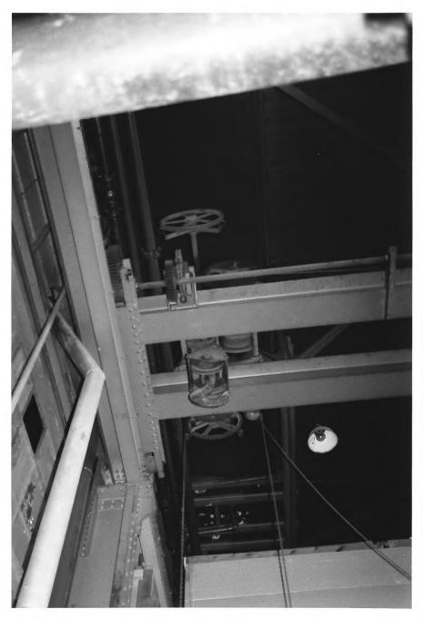
Detail of overhead hoist and steel track for working on diesel generators. Grand Canyon Power House Grand Canvon National Park
