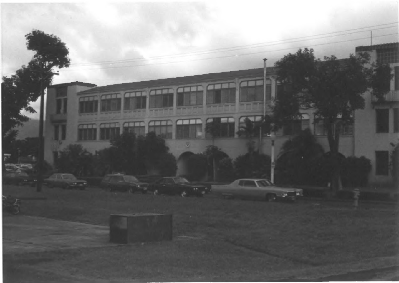
Enlisted men's barracks, Wheeler Air Force Base, 1983.
