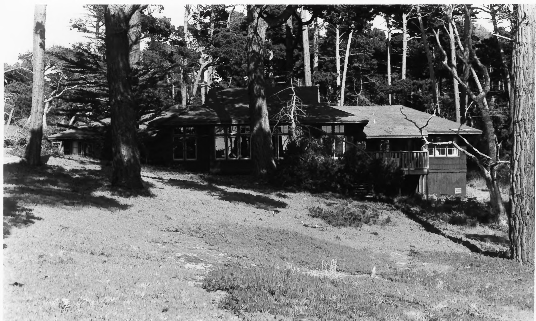
Hilltop (c. 1918), Asilomar Conference Grounds. View looking east from Viewpoint. (Aaron A. Gallup, California Office of Historic Preservation, 1984)
