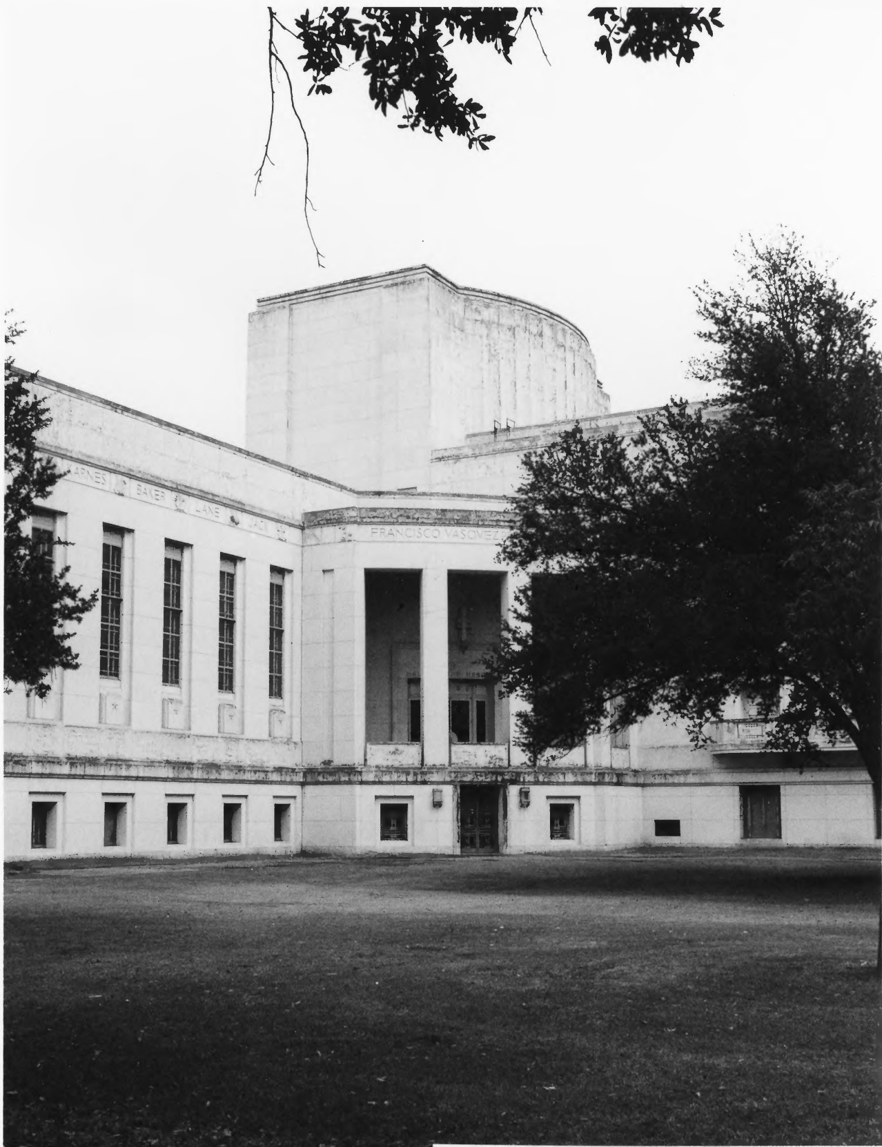
Hall of State, side. (Stephen Snyder, National Park Service, 1985)
