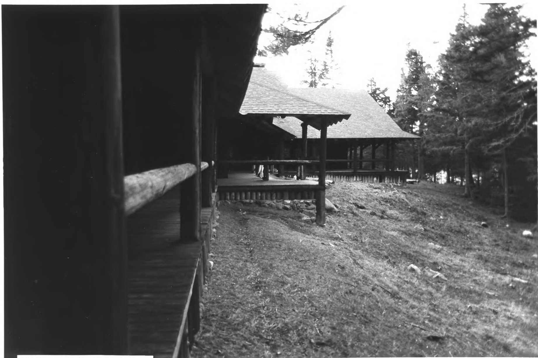
SANTANONI PRESERVE Essex County, New York Lake-facing veranda, looking west Photo by Austin O'Brien, 1994
