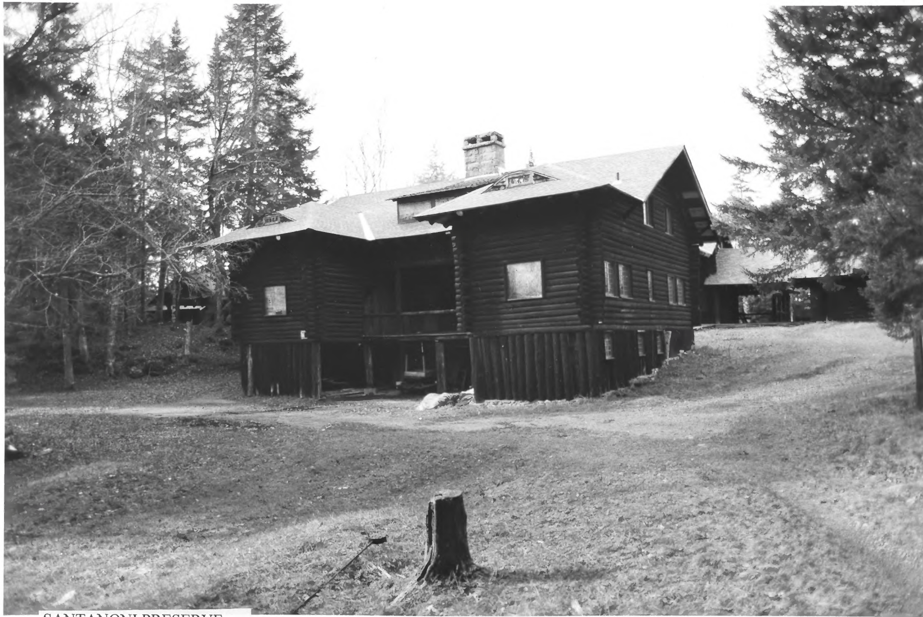
SANTANONI PRESERVE Essex County, New York Kitchen, rear elevation Photo by Austin O'Brien, 1994
