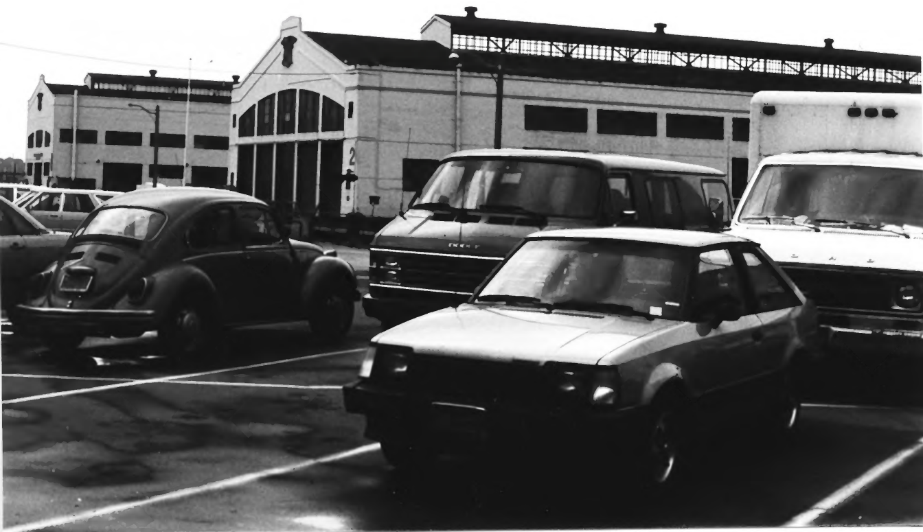
4. Piers 1, on left, and 2, San Francisco Ports of Embarkation. The shed on Pier 2 is the original, permanent shed. Pier 1's shed was reconstructed in the 1930s.
